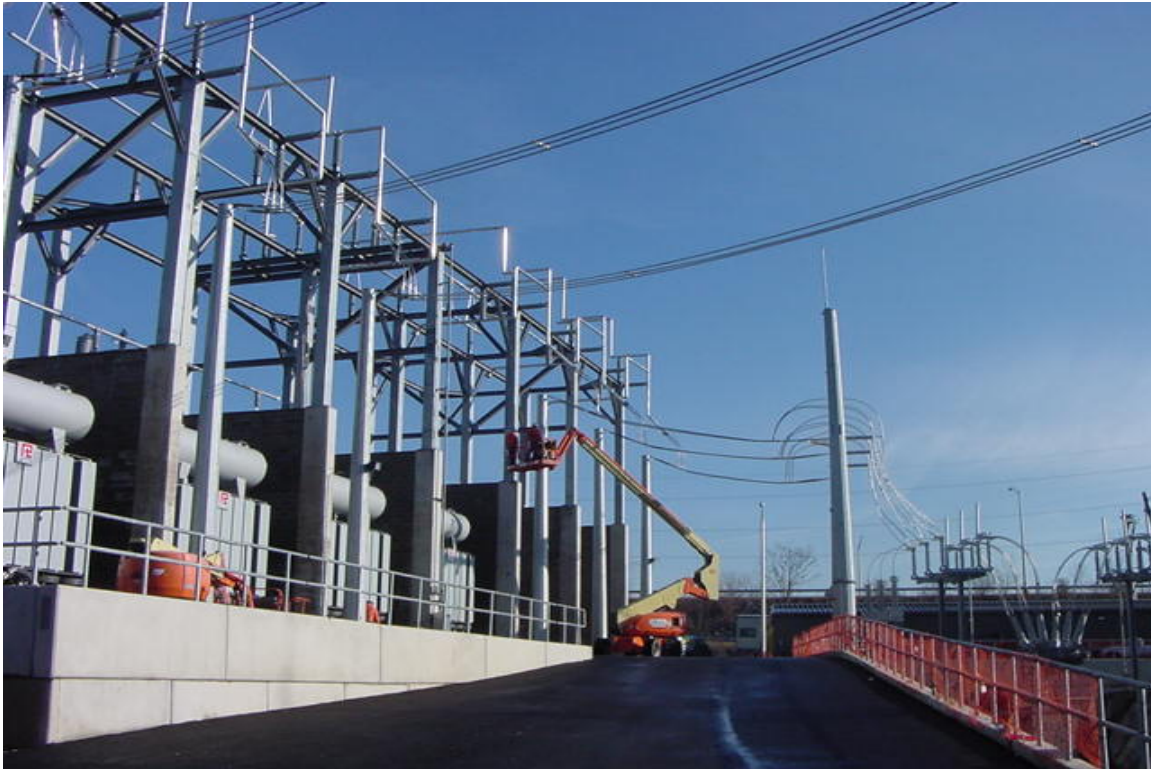
View of work occurring to the structures along the front bays of the GIS building. 1/12/06.
