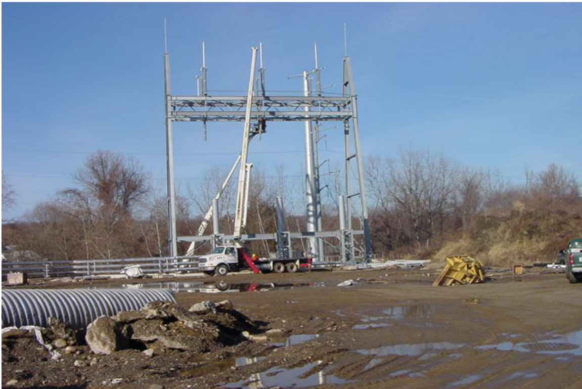
View of the ongoing work on the structures recently installed to the north of the GIS building near the retaining wall. 1/12/06.
