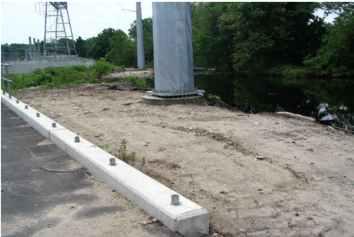
Photo on the left shows the structure near Norwalk Substation. Erosion controls remain in place but the area should be re-vegetated for further stability soon, even if it is only temporarily until the pole is accessed. 6/14/06
