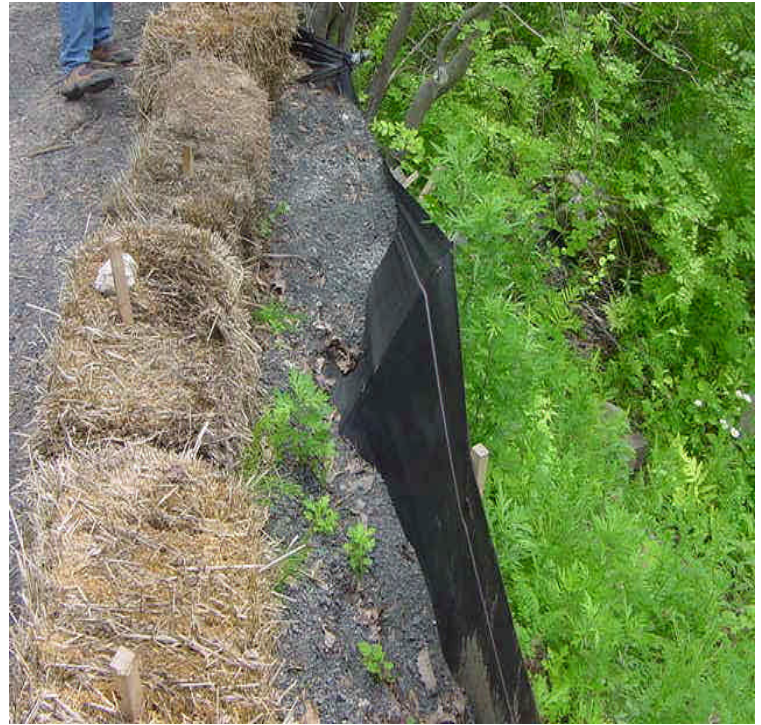
(Composite Section): Photo on the left shows the disturbed area remaining around structure #34 off Gallows Hill. Sediment is beginning to overtop the silt fence again. Photo on the right shows the spot along the Archers Lane ROW where the access road stone overtopped the fence. A new haybale was placed here but stone needs to be pulled back. 6/14/06
