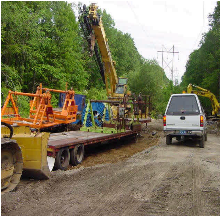
Photo on the left shows the machinery on site to pull wire in the area of John Todd Way. Photo on the right shows the separate contractor (unrelated to the project) placing fill for a driveway in the same area. This contractor is not using erosion controls. 6/14/06.
