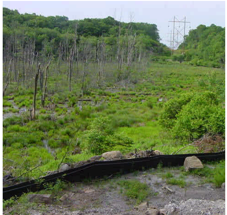
Photo on the left shows the erosion near structure #2. Silt fence was repaired and haybales were placed to reinforce the area. Photo on the right shows where the silt fence was repaired near structure #24. Sediment was also pulled back from the wetland. 6/14/06.
