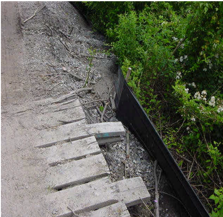
Photo on the left shows where silt fence was overtopped by stone and sediment along a wetland crossing at Kent Rd (south) as a result of the recent rains. The controls here should be repaired.
