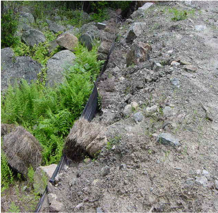
(Composite Section): Photo on the left shows the disturbed area remaining around structure #34 off Gallows Hill. Sediment is beginning to overtop the silt fence again. Photo on the right shows the spot along the Archers Lane ROW where the access road stone overtopped the fence. A new haybale was placed here but stone needs to be pulled back. 6/14/06
