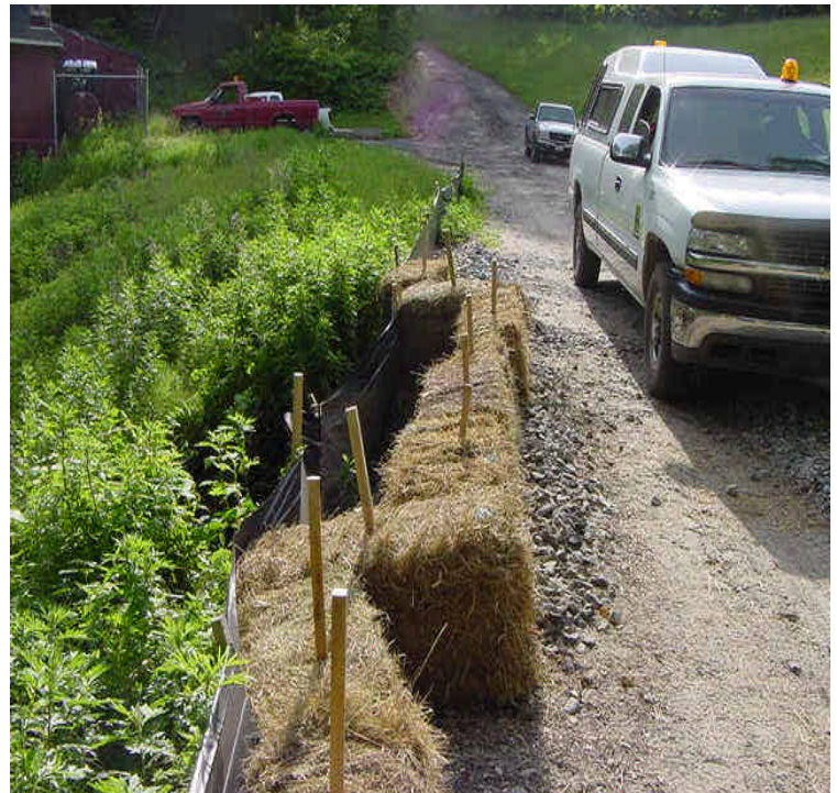
(345kV H-Frame): Photo on the left shows a view of the wetland between structures #10 and #11. Adjacent landowners have reported vehicles here which are not project related. Some silt fence across the access road may help to prevent this. Photo on the right shows haybales installed along the Bethel Reservoir access road. 6/14/06.
