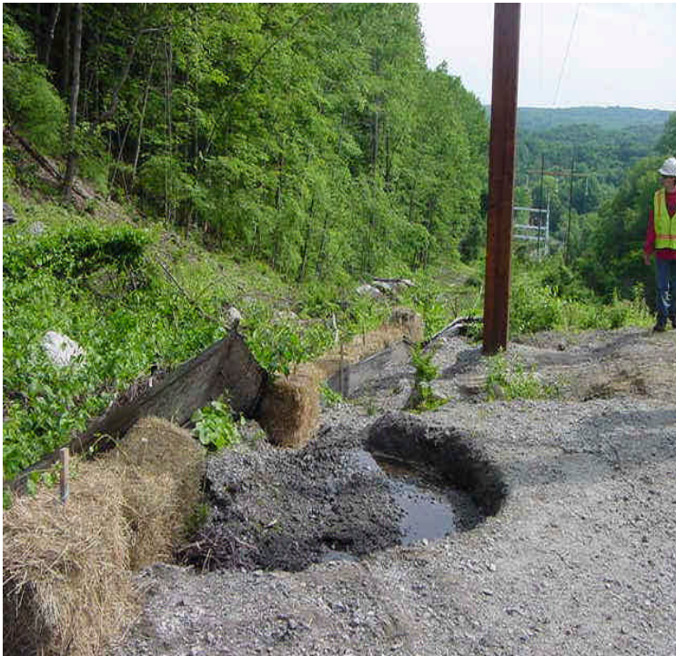
Photo on the left shows the erosion near structure #2. Silt fence was repaired and haybales were placed to reinforce the area. Photo on the right shows where the silt fence was repaired near structure #24. Sediment was also pulled back from the wetland. 6/14/06.
