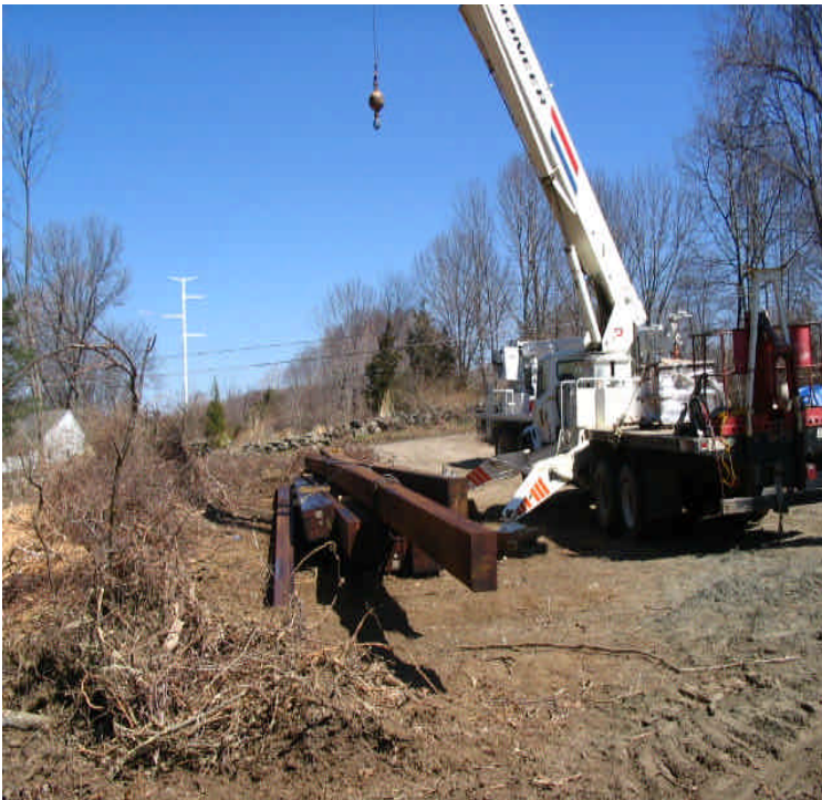
(345kV H-Frame): Photo on the left shows a view of the area near structure #10 where most poles have been removed for installation along the ROW. Photo on the right shows the mats installed at the stream and water main crossing between Poles #10-11 for accessing the remainder of the ROW. Mats were also installed over a 2 nd wet area and controls were installed well. 3/29/06.
