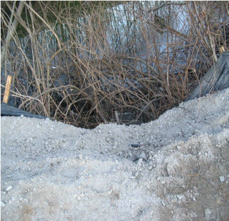
Photo on the left shows where stone dust was pushed over the silt fence. The stone dust should be pulled back and fence repaired ASAP due to proximity of the waterway. The photo on the right shows dirt piled completely over the silt fence. Fence needs repair ASAP, again due to the adjacent wetland. 3/29/06.
