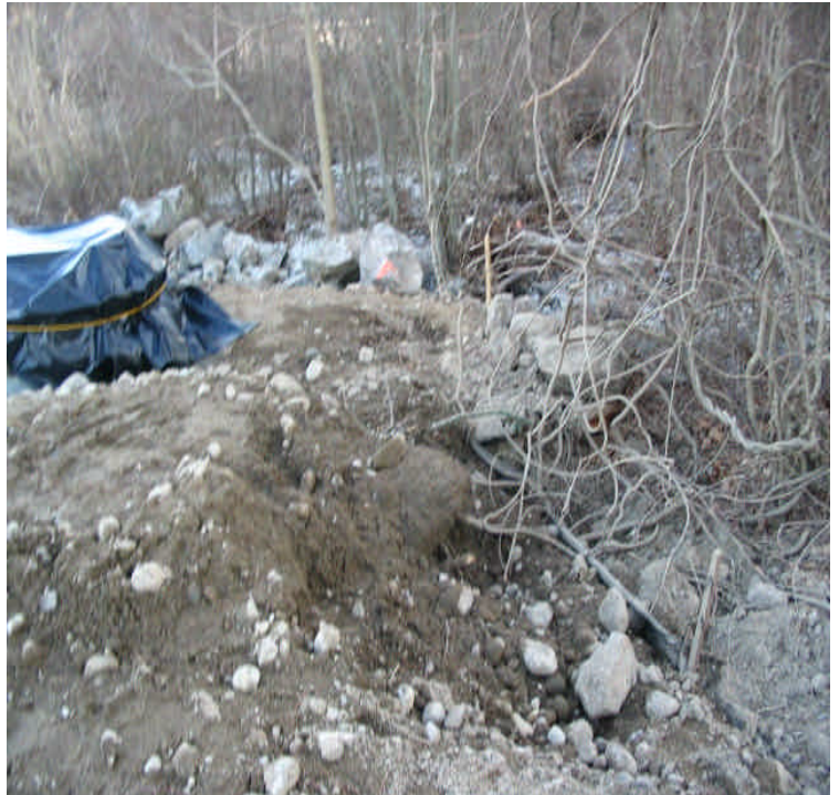
Photo on the left shows where stone dust was pushed over the silt fence. The stone dust should be pulled back and fence repaired ASAP due to proximity of the waterway. The photo on the right shows dirt piled completely over the silt fence. Fence needs repair ASAP, again due to the adjacent wetland. 3/29/06.
