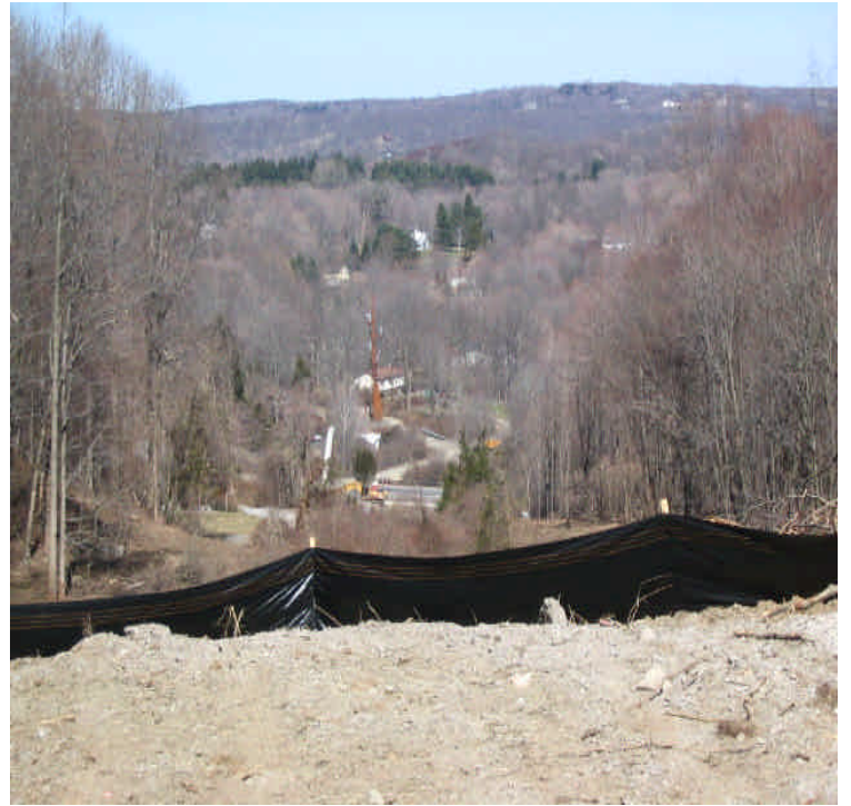
Photo on the left shows the area at structure #9 where the soil stockpile was removed. Silt fence should be maintained here until the area is stabilized. Photo on the right is a view towards Hoyts Hill from structure #2. 3/29/06.
