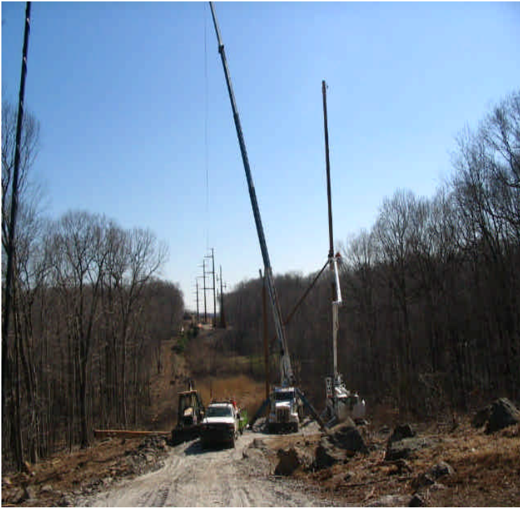
Photo on the left shows structures being installed in the area of Costa Lane. Norwalk Section: Photo on the right shows the stone dust access road to a foundation. A concrete washout was noted here. A containment basin should be set up. 3/29/06
