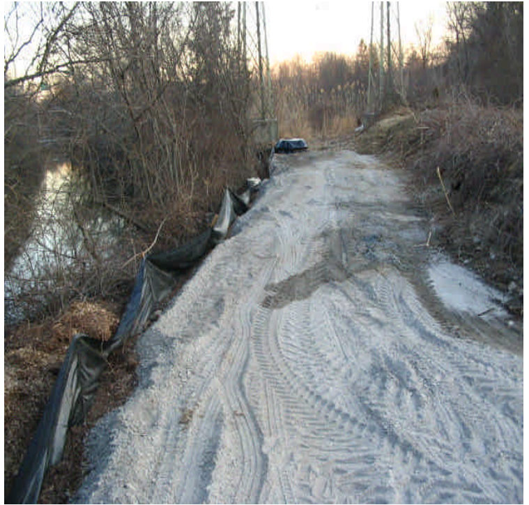
Photo on the left shows structures being installed in the area of Costa Lane. Norwalk Section: Photo on the right shows the stone dust access road to a foundation. A concrete washout was noted here. A containment basin should be set up. 3/29/06
