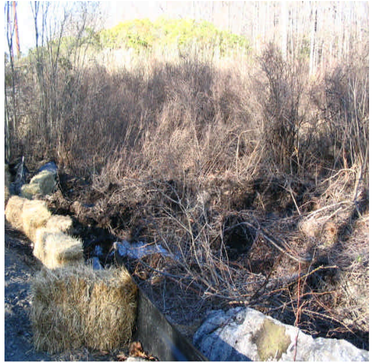
(Composite Section-Archers Lane): Photo on the left shows an overview of the 2 nd crossing at Archers Lane where controls are in good shape. Photo on the right shows where the skidder slipped off the road at the 3 rd crossing and ruts remain in the wetland. 3/29/06.
