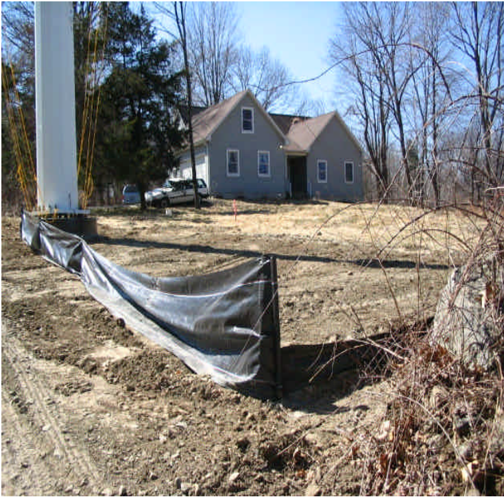
Photo on the left shows the area at structure #9 where the soil stockpile was removed. Silt fence should be maintained here until the area is stabilized. Photo on the right is a view towards Hoyts Hill from structure #2. 3/29/06.
