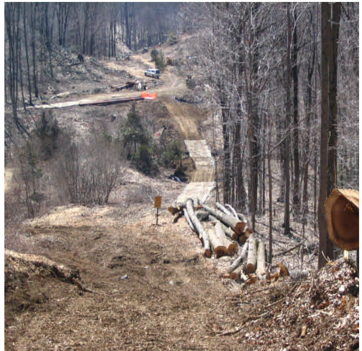
(345kV H-Frame): Photo on the left shows a view of the area near structure #10 where most poles have been removed for installation along the ROW. Photo on the right shows the mats installed at the stream and water main crossing between Poles #10-11 for accessing the remainder of the ROW. Mats were also installed over a 2 nd wet area and controls were installed well. 3/29/06.
