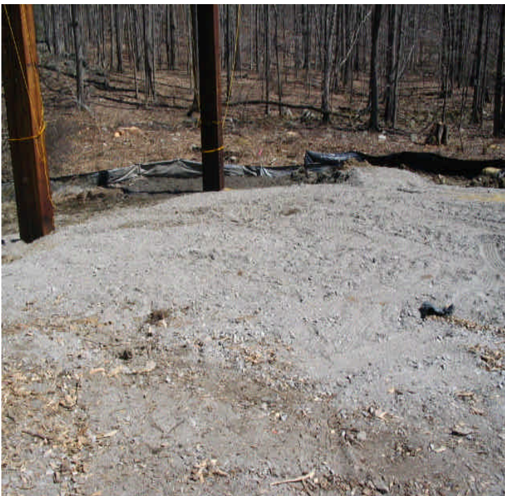
Photo on the left shows the area near structure #6 where the temporary stockpile was removed after pole installation. Remaining sediment will continue to be removed. Photo on the right shows the wetland in this area was not damaged during pole removal and installation. 3/29/06.
