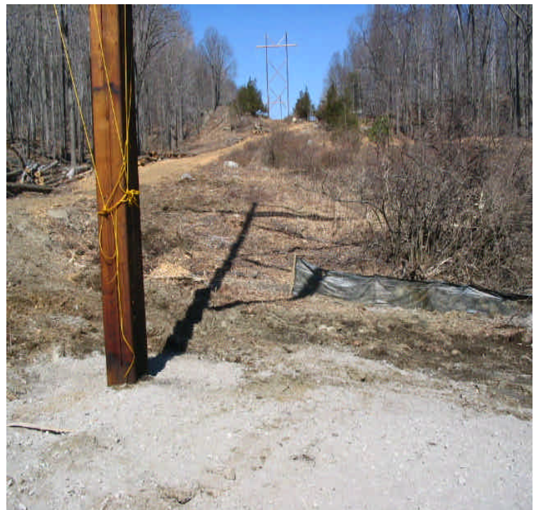
Photo on the left shows the area near structure #6 where the temporary stockpile was removed after pole installation. Remaining sediment will continue to be removed. Photo on the right shows the wetland in this area was not damaged during pole removal and installation. 3/29/06.
