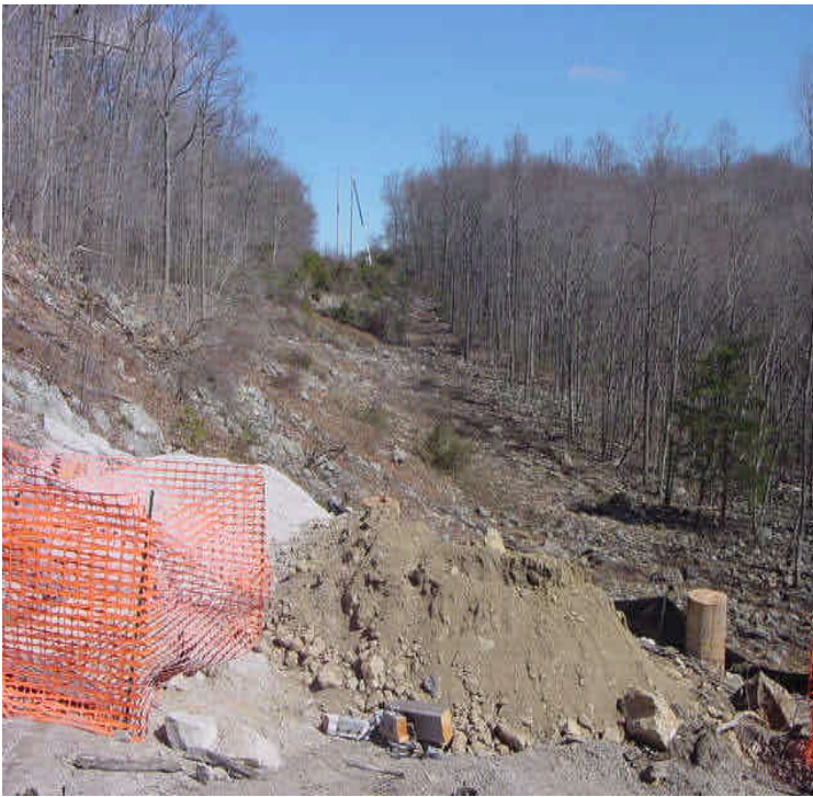
Photo on the left shows the excavation at a pole location off Costa Lane. A structure is being installed in the background of the photo. Photo on the right shows ongoing work at another pole location off Costa Lane. 3/23/06
