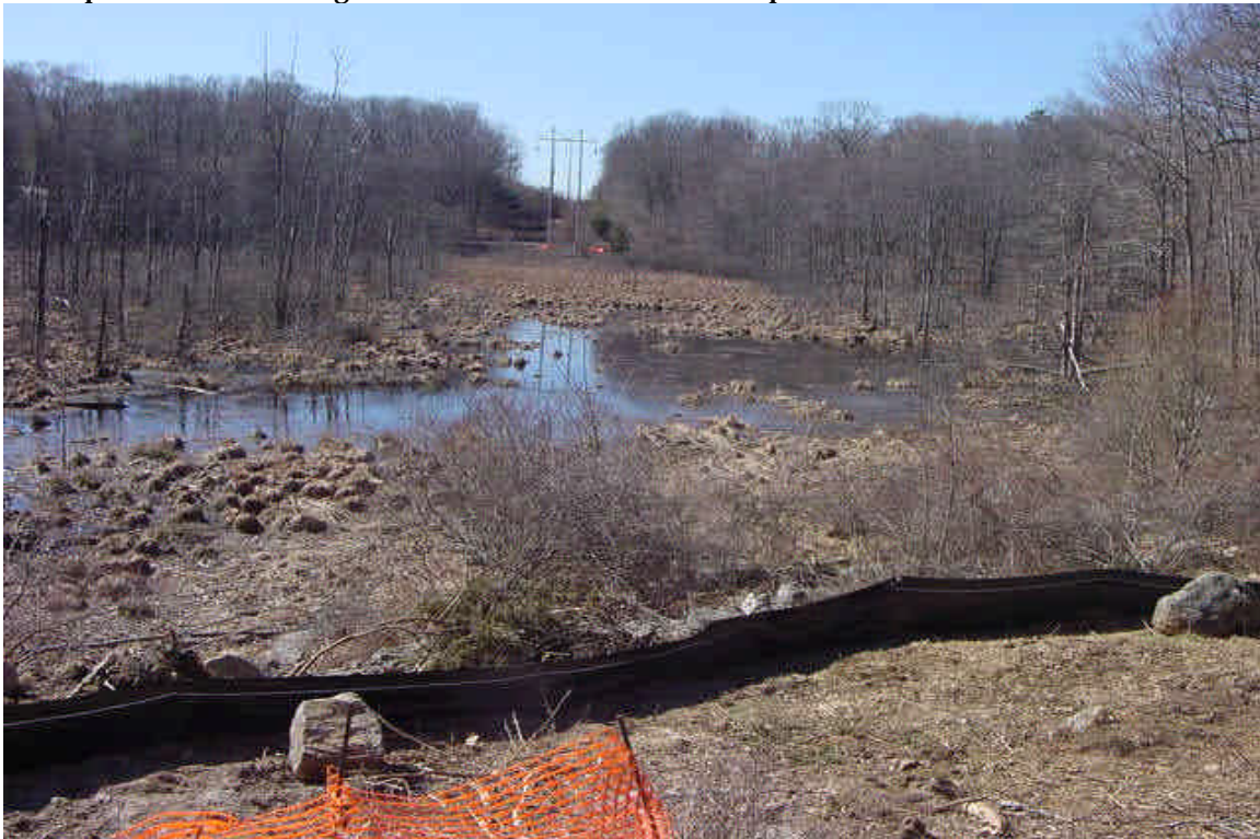
Photo shows a view of the extensive wetland near John Todd Way between poles #24-25. Silt fence is well installed at both sides of the wetland near the pole foundations. 3/23/06
