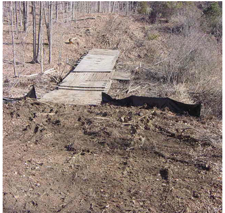
(345kV H-Frame): Photo on the left shows an overview of the Chestnut Ridge Section with several of the new H-frame structures installed. Photo on the right shows the mats installed at the stream and water main crossing between Poles 10-11 for accessing the rest of the ROW. 3/23/06.
