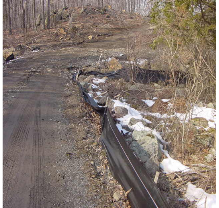
Photo on the left shows the erosion controls near the wetlands at the second structure off Gallows Hill. Sediment has been pushed over them and needs to be pulled back. Photo on the right shows the wetland crossing at the same location where silt fence is down. 2/22/06
