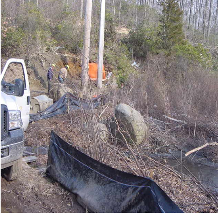
Photo on the left shows silt fence which has been installed at pole #19 now that foundation work is beginning here. Photo on the right shows the view along the access road in the Bethel Reservoir section with new wood chips in place to help stabilize. 2/22/06
