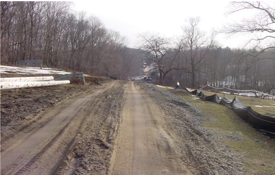
View of the access road and erosion controls near pole #7. Some repairs to the silt fence were recommended here. 2/22/06
