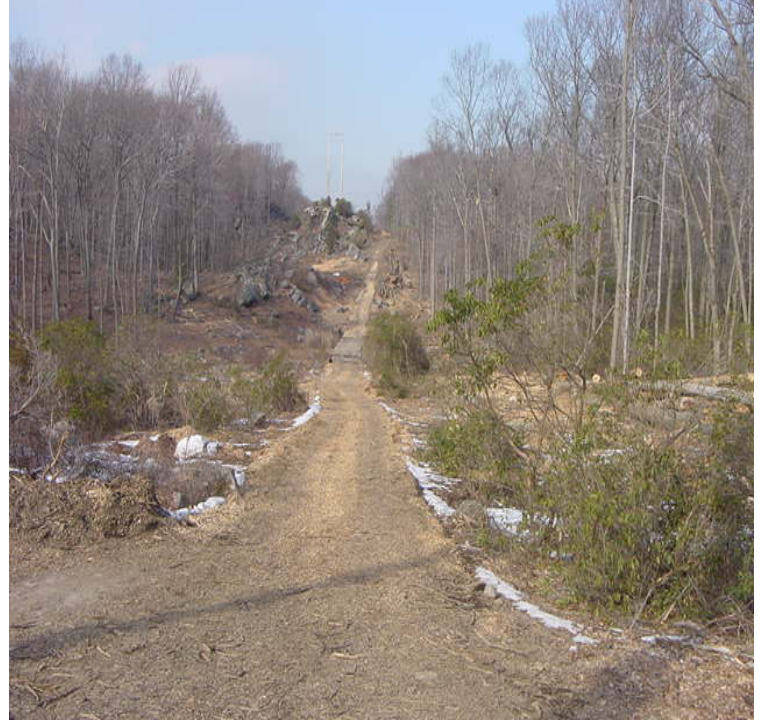
Photo on the left shows silt fence which has been installed at pole #19 now that foundation work is beginning here. Photo on the right shows the view along the access road in the Bethel Reservoir section with new wood chips in place to help stabilize. 2/22/06
