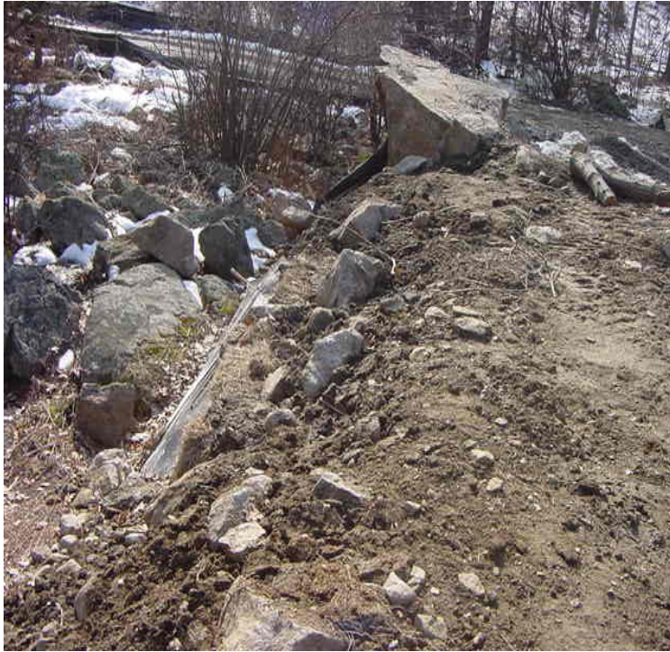
Photo on the left shows the erosion controls near the wetlands at the second structure off Gallows Hill. Sediment has been pushed over them and needs to be pulled back. Photo on the right shows the wetland crossing at the same location where silt fence is down. 2/22/06
