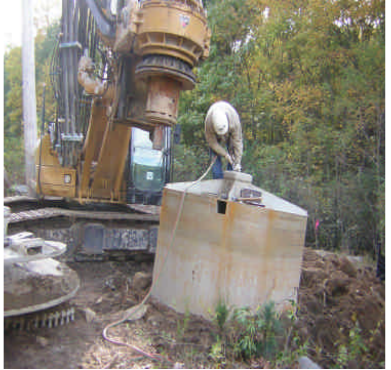
Photo on the left shows a view of the excavation for the next structure foundation moving south along the ROW. The area here was all upland and controls were well in place. Photo on the right shows work at a caisson closer to Archers Lane along the ROW. (10/19/05)
