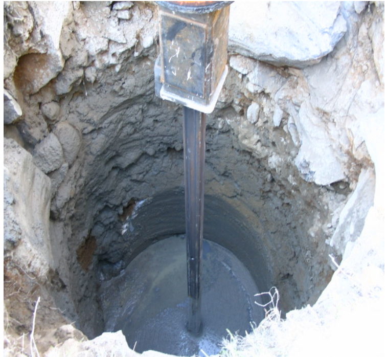
hole for the caisson/foundation with the thick muddy water to be removed. The stone dust created by the drilling accounts for the color. (10/5/05)
