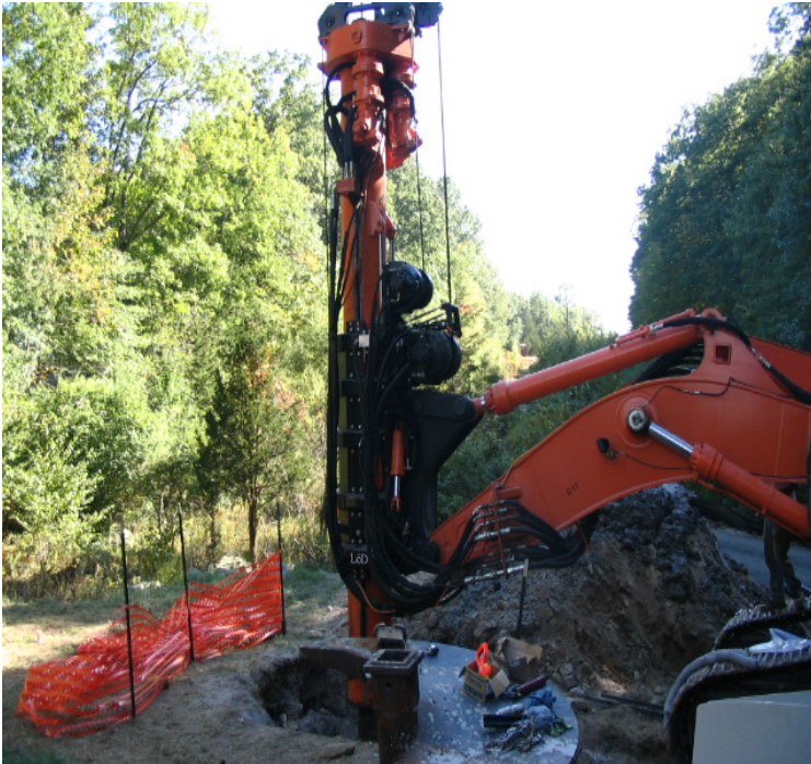
hole for the caisson/foundation with the thick muddy water to be removed. The stone dust created by the drilling accounts for the color. (10/5/05)
