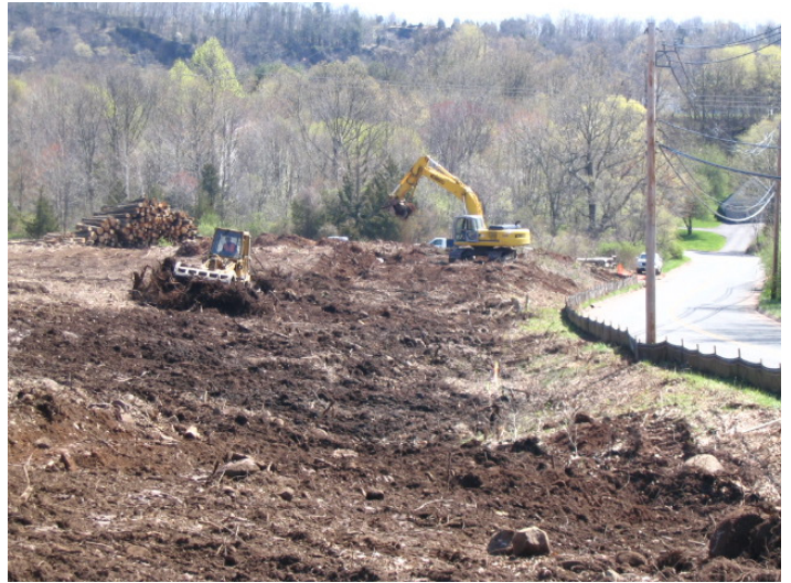
Silt fence being installed on east side of site
