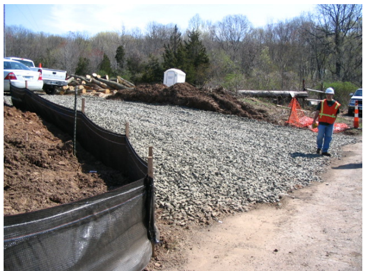
Crushed stone construction entrance on Carpenter Lane
