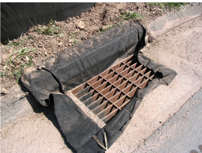
Catch basin on Carpenter Lane protected with silt sack
