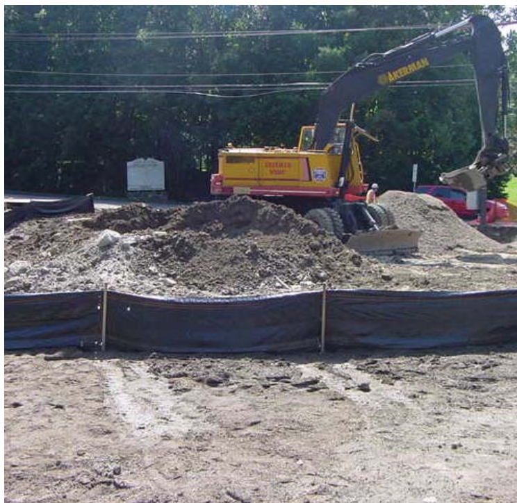
Photo on the left shows the grading and backfill work at the jacking pit at the jack & bore. Good silt fence is in place. Photo on the right shows the down-gradient line of silt fence in good shape. 9/7/06
