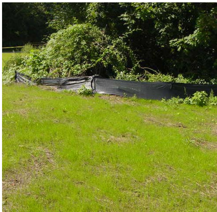
345kV XLPE: Both photos show the restored area in the ball park and near the streambank. Grass growth is returning and silt fence is in good shape. Continue to monitor. 9/7/06
