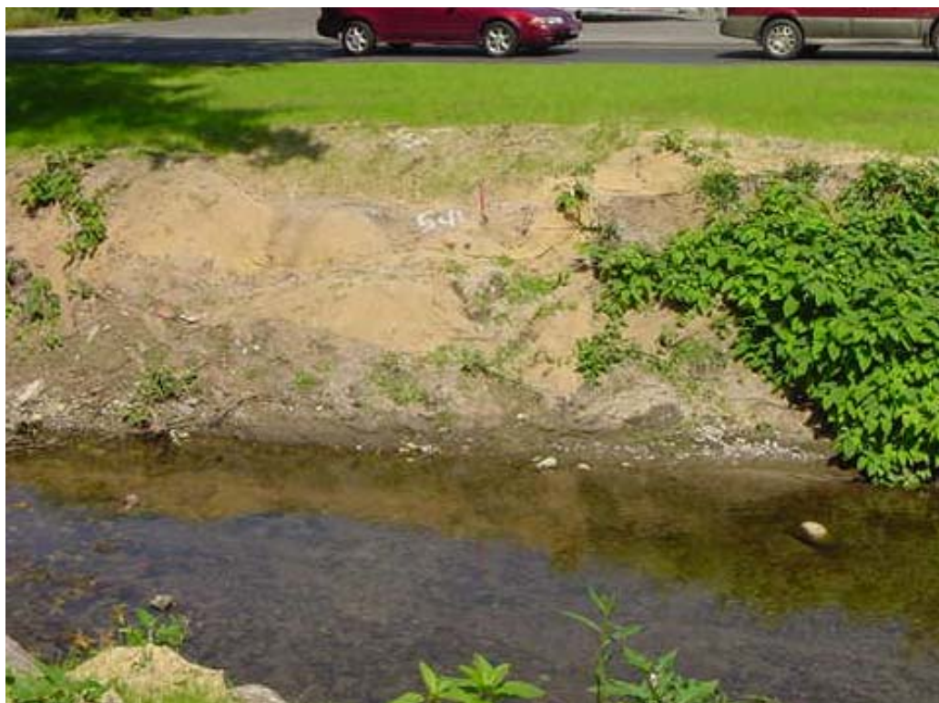
Photo shows vegetative growth returning in portions along the streambanks with the erosion control blankets in place. Some areas remain sparse and could use additional cover. 9/7/06
