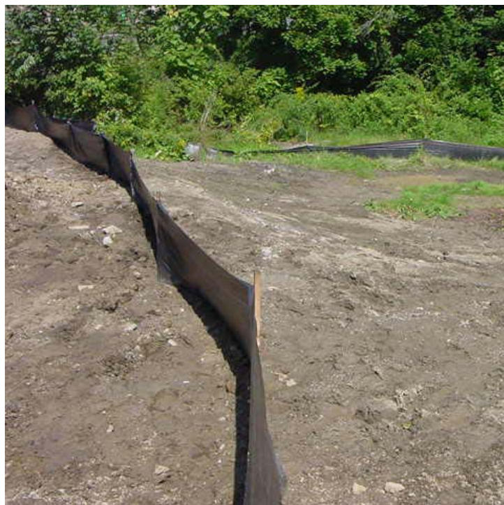
Photo on the left shows the grading and backfill work at the jacking pit at the jack & bore. Good silt fence is in place. Photo on the right shows the down-gradient line of silt fence in good shape. 9/7/06
