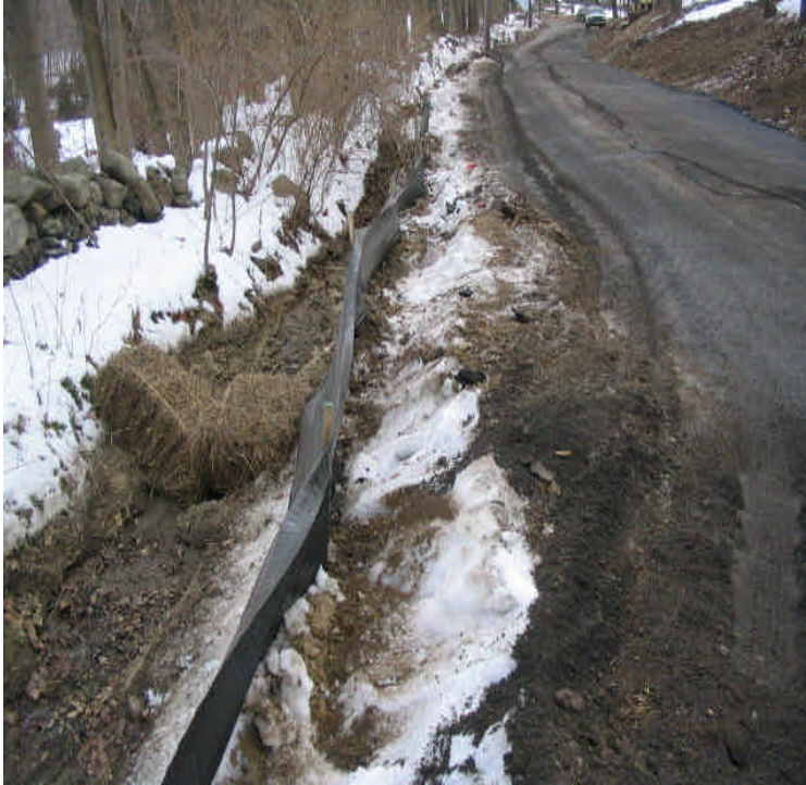
345kV (Umpawaug Rd Daywork): Silt fence and haybales have been installed along swales and wetland areas near the Diamond Hill Rd. intersection. Some sedimentation buildup was noted near the controls. It should be removed if possible. 12/22/05
