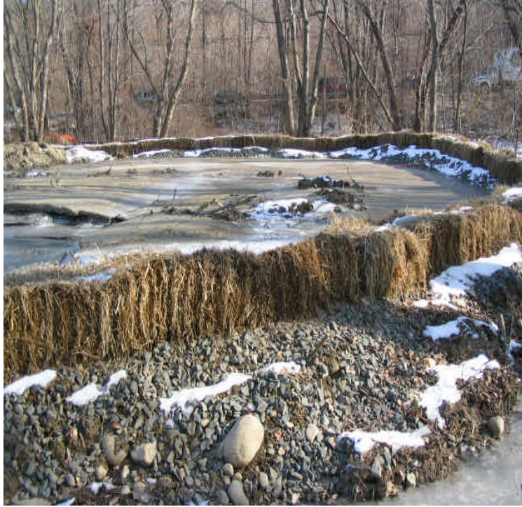
345kV (HDD School Rd.) Both photos show views of the settling basin, still receiving turbid water and mud. No excavation or cleaning of he basin has occurred as discussed. 12/22/05
