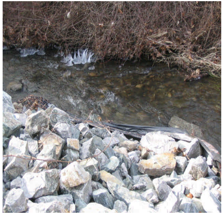
345kV (Georgetown Deli Jack and Bore): Photo on the left shows the receiving pit side where additional sandbags had been installed following the recent rain and flood event. Photo on the right shows where the silt fence at the dewatering outlet had been washed down. The stream was slightly turbid at this inspection. 12/22/05
