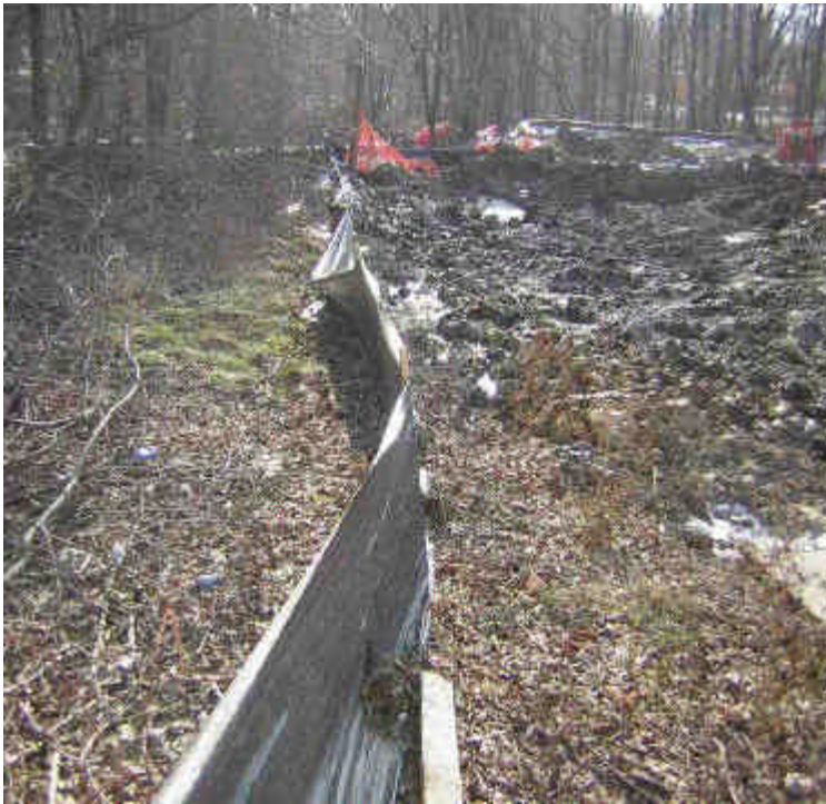
Photo on the left shows the perimeter silt fence and disturbed soil surface along the east of the site. Additional stability is needed here to prevent further disturbance during equipment access. The photo on the right shows a small spill (likely of fuel) near the tank on site. 12/22/05
