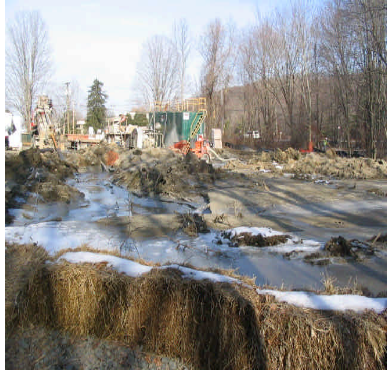
345kV (HDD School Rd.) Both photos show views of the settling basin, still receiving turbid water and mud. No excavation or cleaning of he basin has occurred as discussed. 12/22/05
