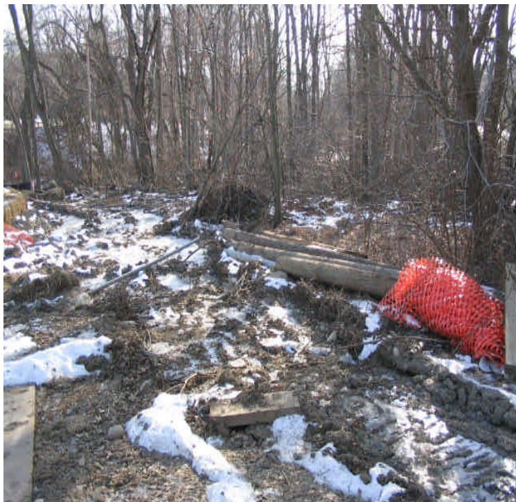
Photo on the left shows some disturbed areas to the west of the basin while the photo on the right is a view of the work area and associated disturbed soil. Any equipment access to or around the basin should be done on mats preferably, or temporary stone on fabric to prevent further disturbance or ruts. 12/22/05
