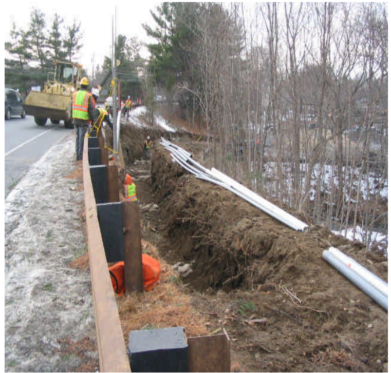
345kV (Rt 107): Photo on the left shows a view of where pipe is being installed above a bridge over the Norwalk River. Sit fence is in place at this time. Photo on the right shows a view of this work from the roadway. 12/22/05
