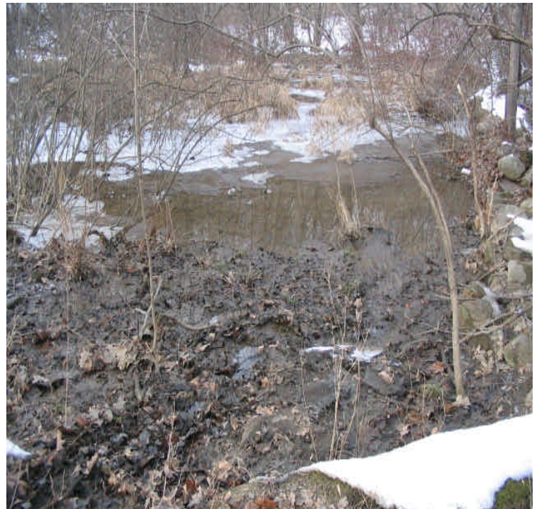
Both photos show a view of where sediment and turbid water migrated through a swale to the adjacent wetland near the work at #79 Umpawaug Rd. The inlet to this swale did have haybales installed but it wasn't enough prevent the sedimentation. 12/22/05
