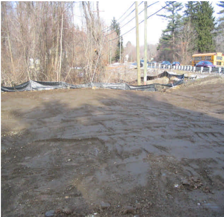
345kV (Wilton High School J&B): Photo on the left shows where the old settling basin has been filled in and the area regraded. Photo on the right shows a spot where the remaining erosion controls are lacking. This fence should be repaired as soon as possible. 12/22/05
