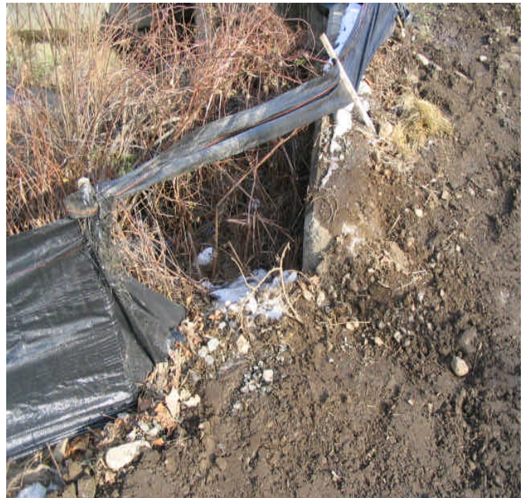
345kV (Wilton High School J&B): Photo on the left shows where the old settling basin has been filled in and the area regraded. Photo on the right shows a spot where the remaining erosion controls are lacking. This fence should be repaired as soon as possible. 12/22/05
