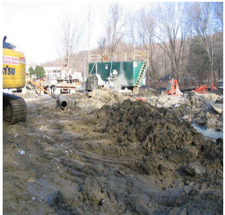
Photo on the left shows some disturbed areas to the west of the basin while the photo on the right is a view of the work area and associated disturbed soil. Any equipment access to or around the basin should be done on mats preferably, or temporary stone on fabric to prevent further disturbance or ruts. 12/22/05
