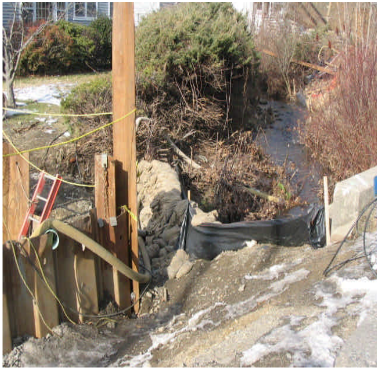
345kV (Georgetown Deli Jack and Bore): Photo on the left shows the receiving pit side where additional sandbags had been installed following the recent rain and flood event. Photo on the right shows where the silt fence at the dewatering outlet had been washed down. The stream was slightly turbid at this inspection. 12/22/05
