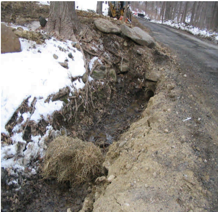
345kV (Umpawaug Rd Daywork): Silt fence and haybales have been installed along swales and wetland areas near the Diamond Hill Rd. intersection. Some sedimentation buildup was noted near the controls. It should be removed if possible. 12/22/05
