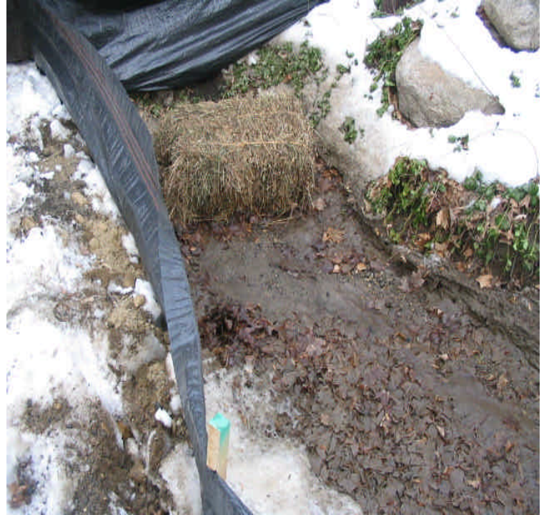
345kV (Umpawaug Rd Daywork): Silt fence and haybales have been installed along swales and wetland areas near the Diamond Hill Rd. intersection. Some sedimentation buildup was noted near the controls. It should be removed if possible. 12/22/05
