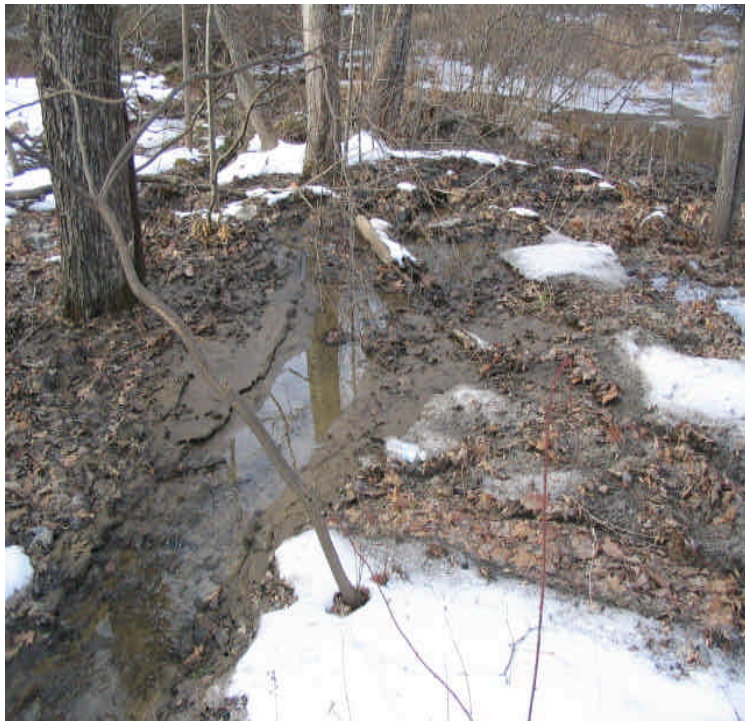
Both photos show a view of where sediment and turbid water migrated through a swale to the adjacent wetland near the work at #79 Umpawaug Rd. The inlet to this swale did have haybales installed but it wasn't enough prevent the sedimentation. 12/22/05
