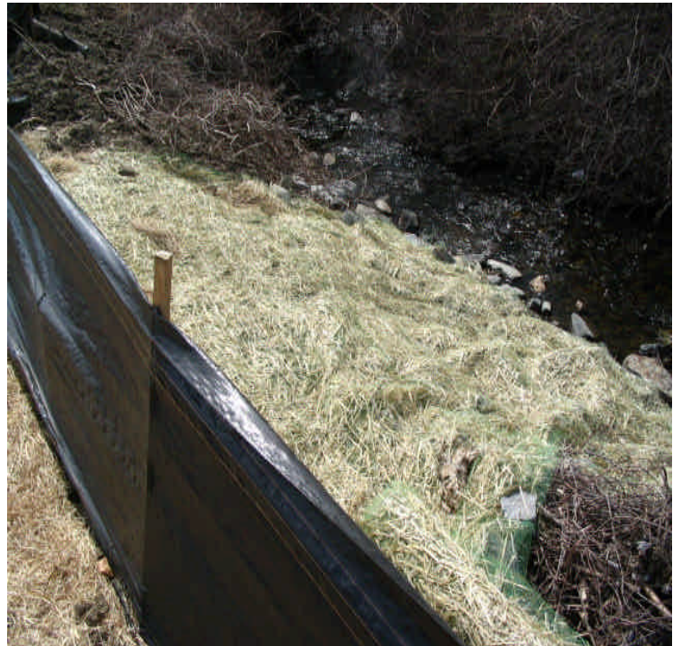
345kV (Georgetown Deli) Photo on the left shows where the small stockpile was removed from the lot. Photo on the right shows the bank controls well in place. 4/12/06
