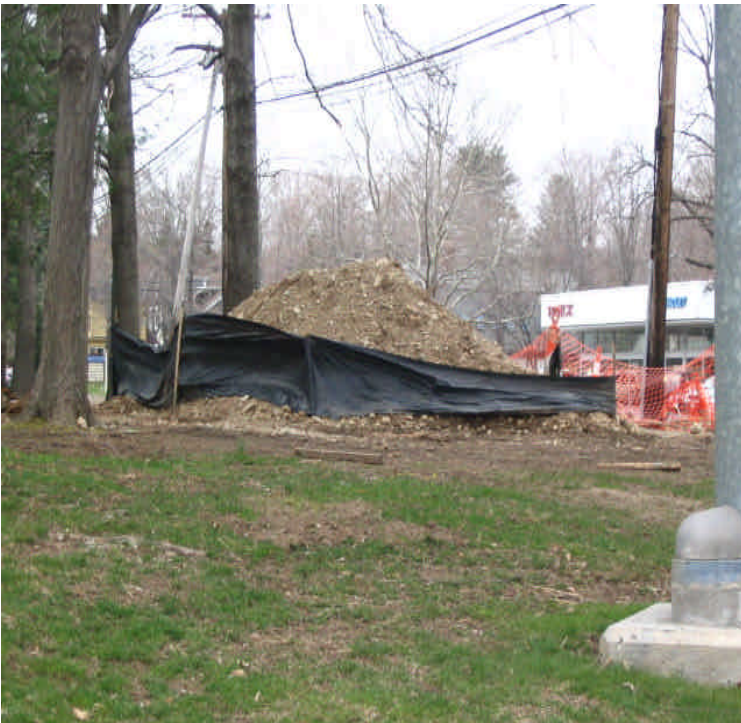
Photo on the left shows silt fence up at the stockpile near the Wilton Corporate Park but it was not toed in. Photo on the right shows the perimeter of Norwalk Junction where 345kV trenching occurred several weeks ago. The resulting stockpiles and excavations were effectively backfilled. 4/12/06
