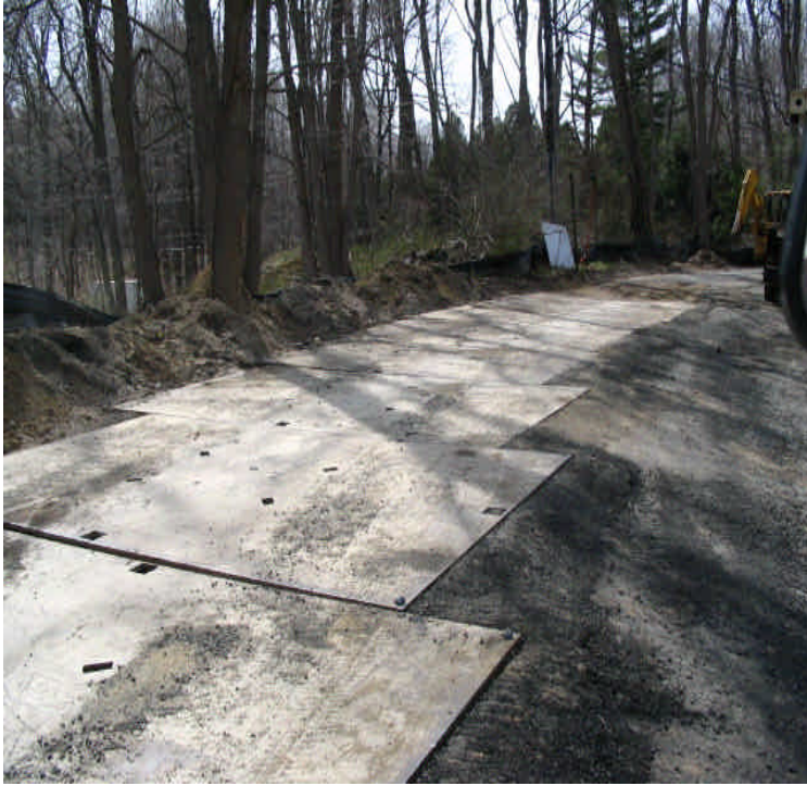
345kV (Diamond Hill-Umpawaug): Photo on the left shows road plate/trench covers on Diamond Hill Rd. Adjacent erosion controls will need to be toed in along the road due to wetlands in close proximity. Photo on the right shows work at the Umpawaug Rd. intersection. 4/12/06
