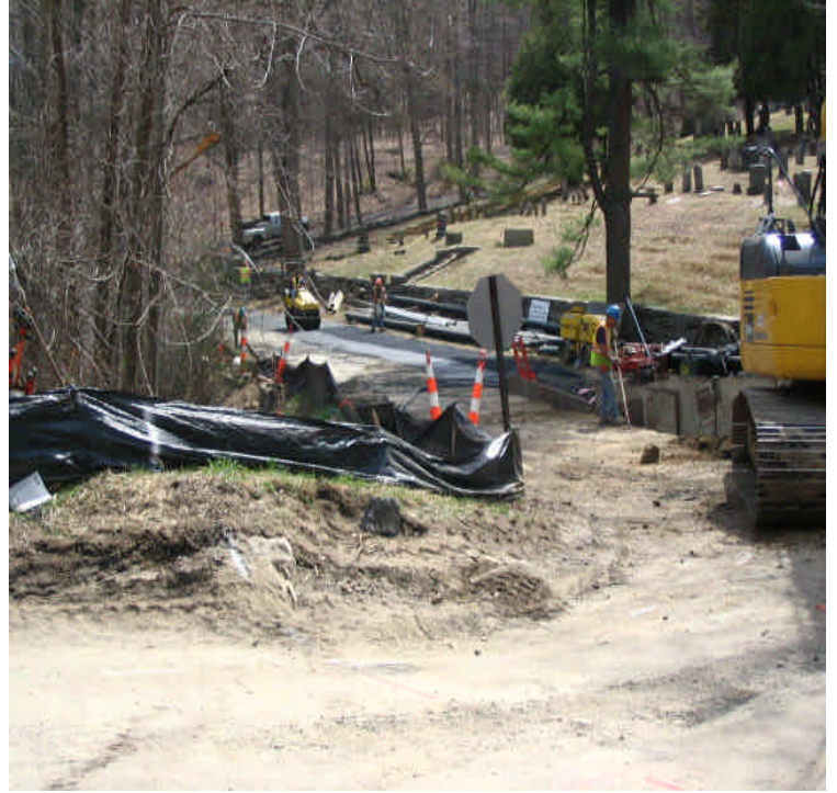
345kV (Diamond Hill-Umpawaug): Photo on the left shows road plate/trench covers on Diamond Hill Rd. Adjacent erosion controls will need to be toed in along the road due to wetlands in close proximity. Photo on the right shows work at the Umpawaug Rd. intersection. 4/12/06
