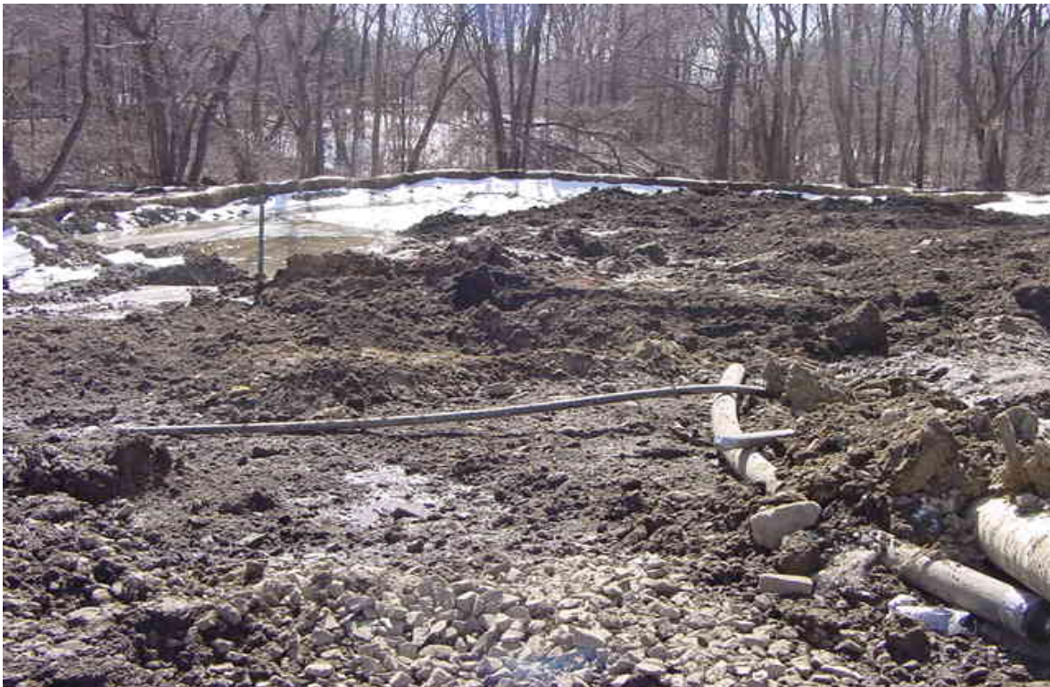
The drill equipment has demobilized and the basin is in the process of being filled in and graded as a temporary stabilization measure. After trenching connects to this area, the soil surface should be revegetated and restored. 3/9/06
