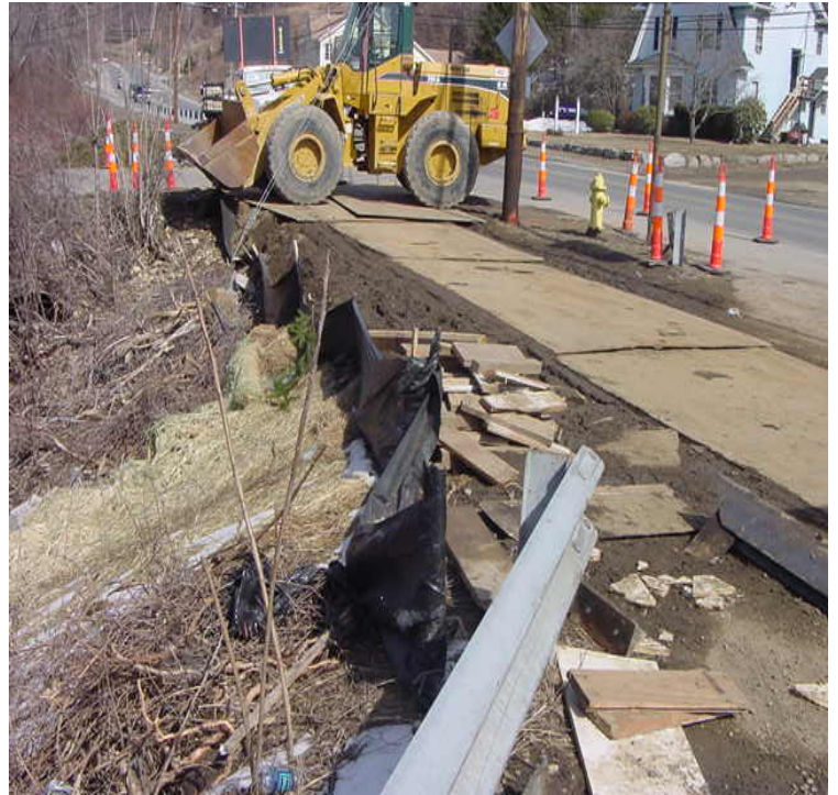
345kV (Rt 107) Photo on the left shows the Georgetown Deli with jute netting well in place along the bank. Photo on the right shows trenching along this area to connect in with the jack and bore. The silt fence needs repair in one area here. 3/9/06
