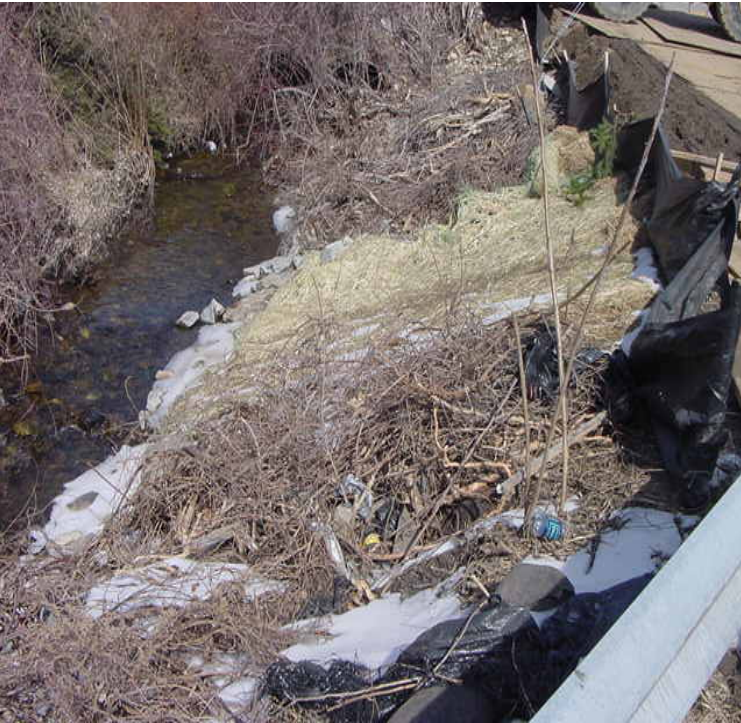
345kV (Rt 107) Photo on the left shows the Georgetown Deli with jute netting well in place along the bank. Photo on the right shows trenching along this area to connect in with the jack and bore. The silt fence needs repair in one area here. 3/9/06
