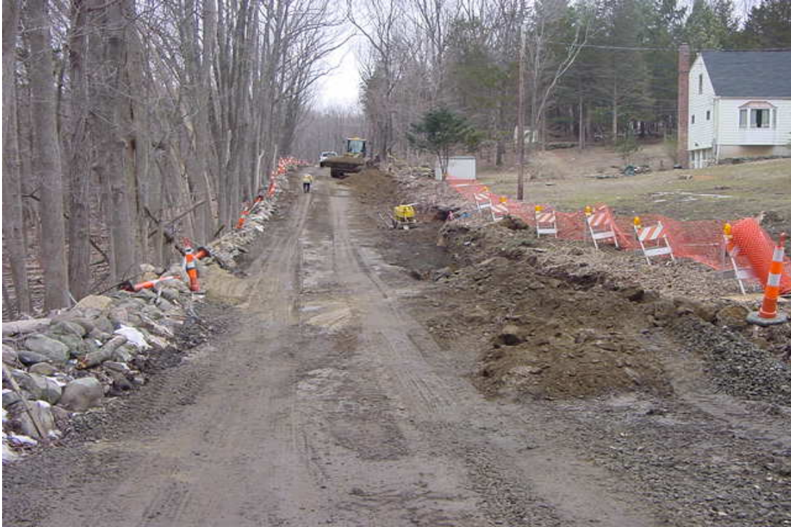
345kV (Archers Lane): Crews were backfilling the 345kV trenchwork along the access drive into the Archers Lane station. The site remains well contained at this time. Watch sediment along the stonewall as wetlands are located beyond it. 3/9/06
