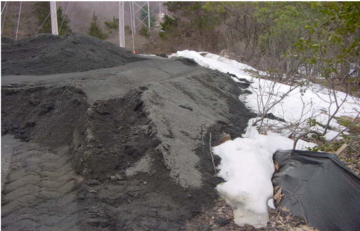
View of a stockpile of flowfill located adjacent to the drive and at the top of a slope leading to wetland. A silt fence was suggested due to its proximity to the slope. 3/9/06
