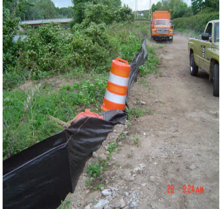
115kV (Broad Street and ROW): The photo on the left shows the corner edge of silt fence near the foundations at the substation which should be repaired. Photo on the right shows a spot along the ROW where the fence should be righted. (9/29/05)
