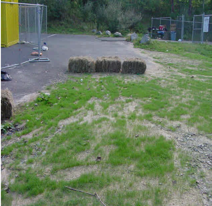
115kV (Bethel Ed. Park): Photo on the left shows haybale check dams placed in an attempt to slow stormwater flow to the ROW. The photo on the right shows the good grass growth at the northern end of the ROW. (9/29/05)
