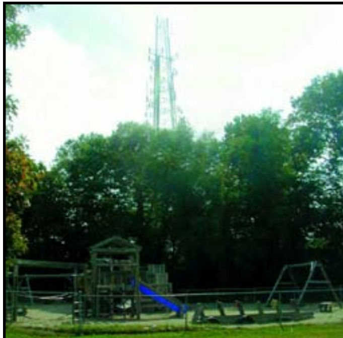
Figure-22. 1320 Chopsey Hill Road in Bridgeport, CT. Photograph taken in October of 2006.
