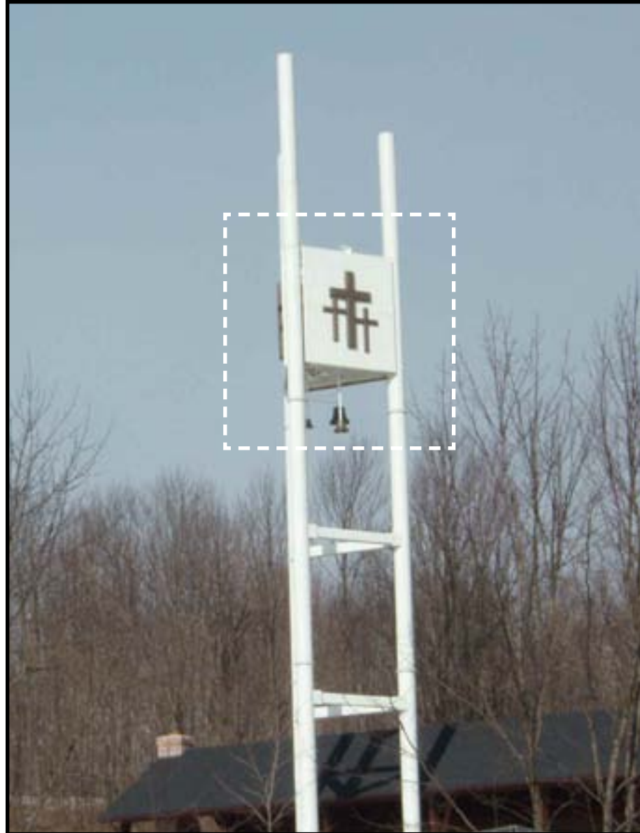
Figure-25. A 125-foot telecommunications facility disguised as a bell tower located at the Harvest Baptist Church at 1440 Litchfield Turnpike in New Hartford, CT. Photographed in February of 2007.
