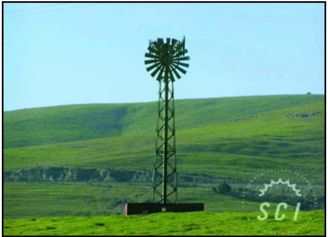
Figure-36. Betteravia Properties in Santa Maria, CA. The structure is 50 feet tall. Antennas are located at 48 feet agl.
