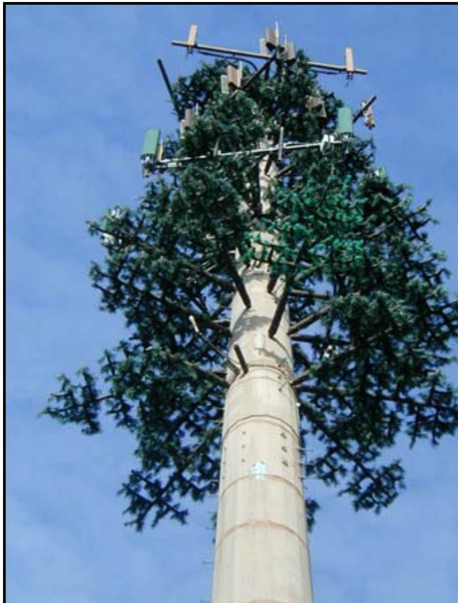
Figure-23. A 120-foot telecommunications facility, disguised as a tree, located at 477 Route 7 in Sharon, CT. Photographed in January of 2007.
