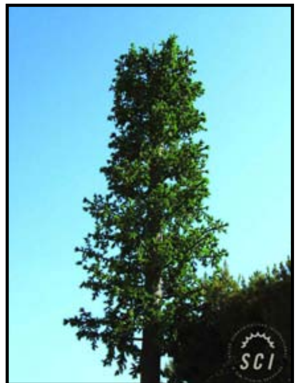
Figure-31. Pacifica Mormandie in Torrance, CA. The structure is 62 feet tall. Antennas are located at 55 feet agl.
