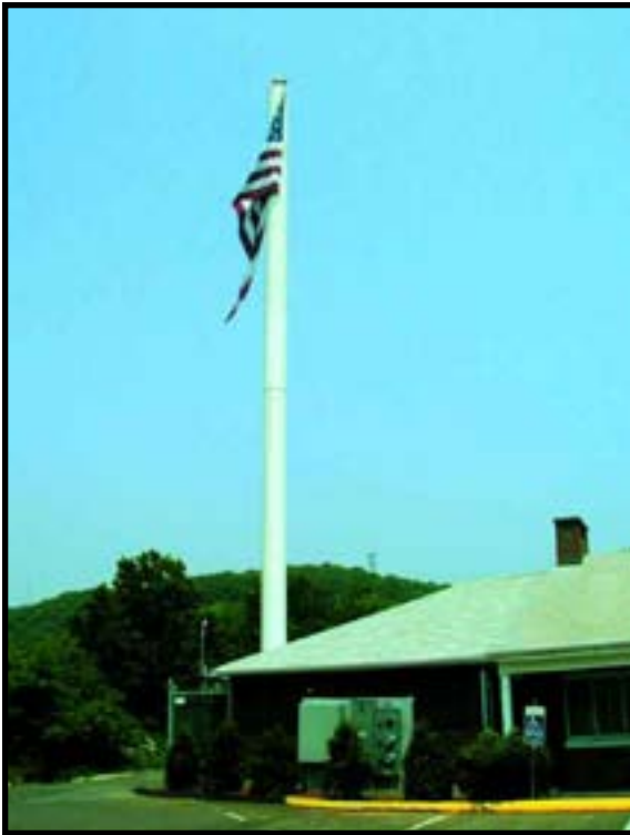
Figure-32. 100 Pond Lily Avenue in New Haven, CT. Antennas are located within the flagpole structure and equipment is housed within a brick façade that matches the building. Photograph taken in June of 2006.
