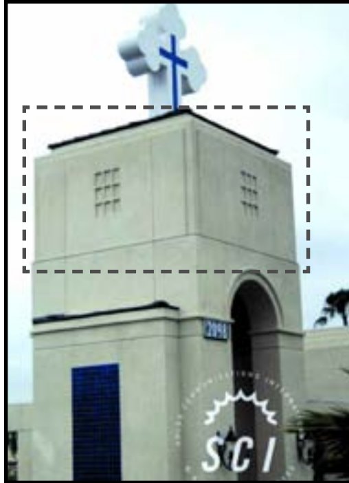
Figure-57. St. George Church Cross in Upland, CA. The structure is 35 feet tall. The top of the antennas extend to 34.5 feet agl.
