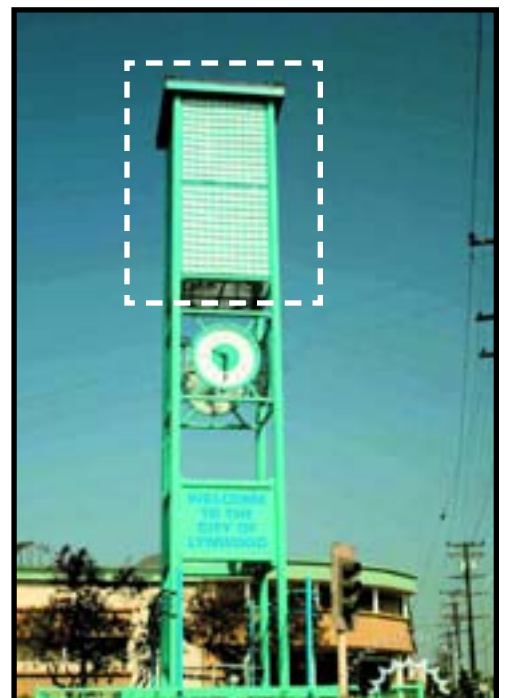
Figure-38. City of Lynwood, CA. Dimensions of the structure are 60 feet tall by 8 feet wide.
