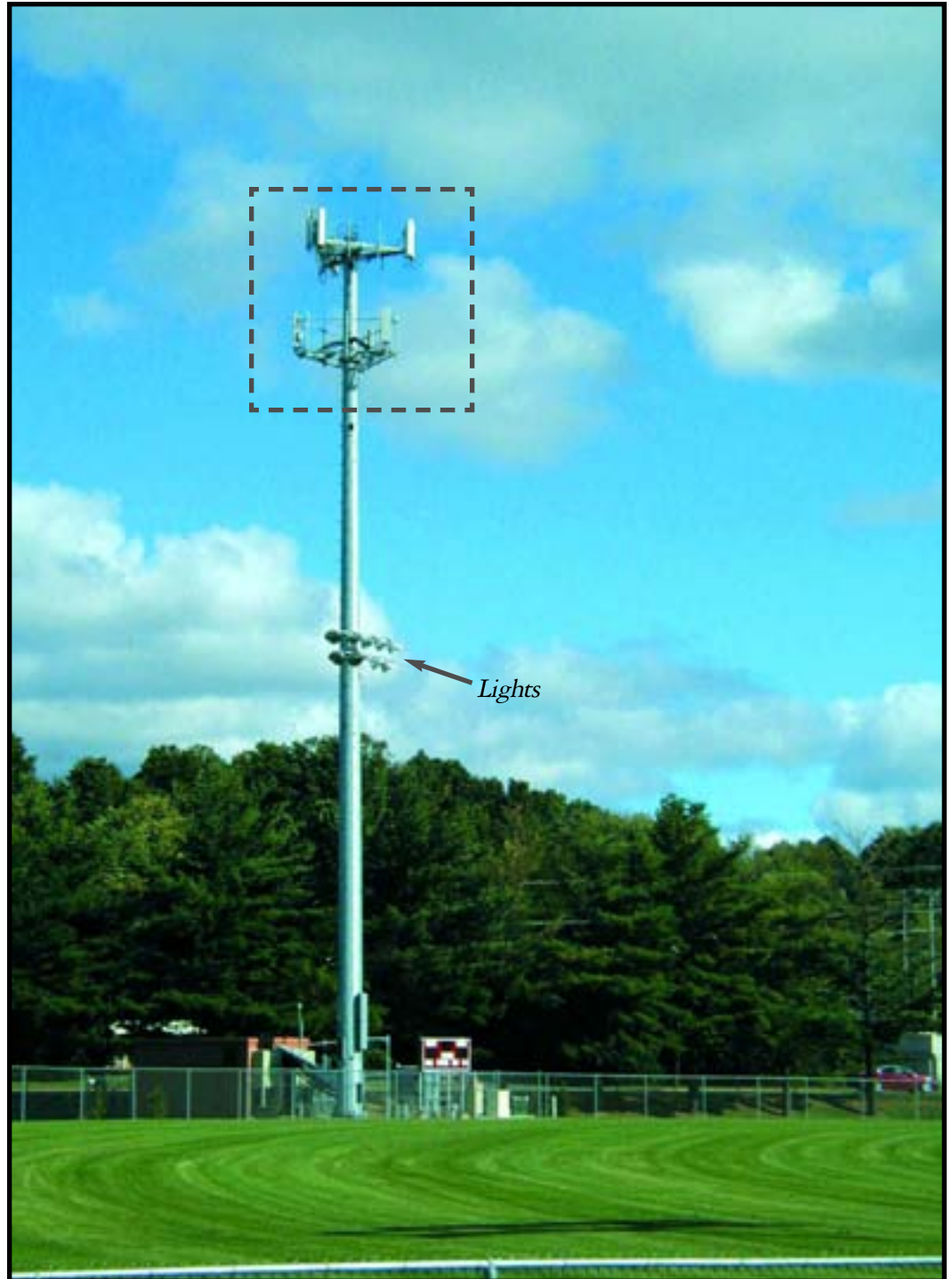
Figure-15. Park lights share a structure with wireless telecommunications antennas at Chelsey Park in New Britain, CT. Photograph taken in September of 2006.
