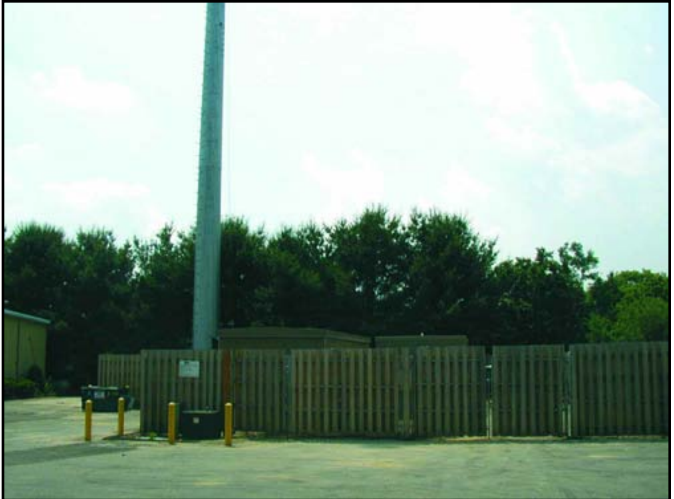
Figure-66. 1725 Stafford Road in Mansfield, CT. Photograph taken in June of 2004.
