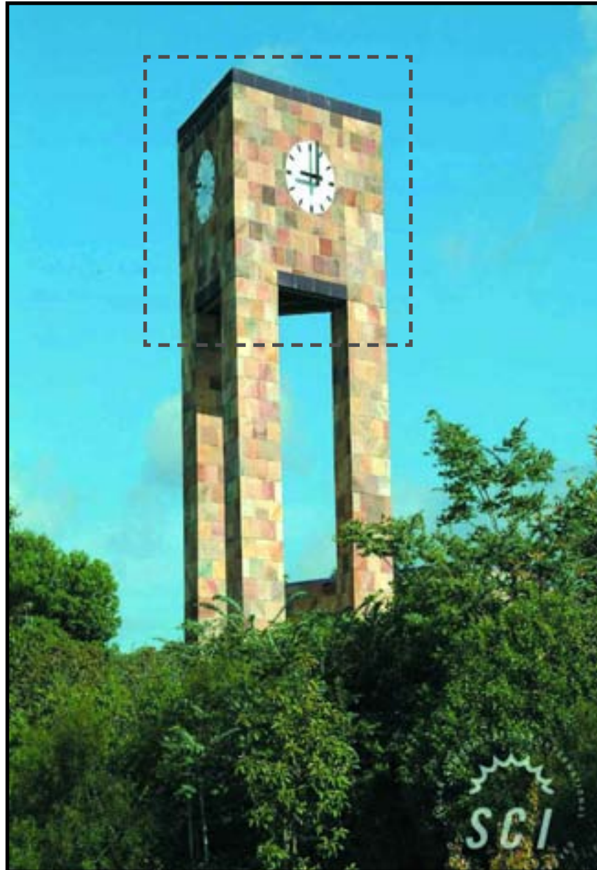
Figure-34. Vista, CA. The structure is 45 feet tall. Antennas are located at 41.5 feet agl and 35 feet agl.
