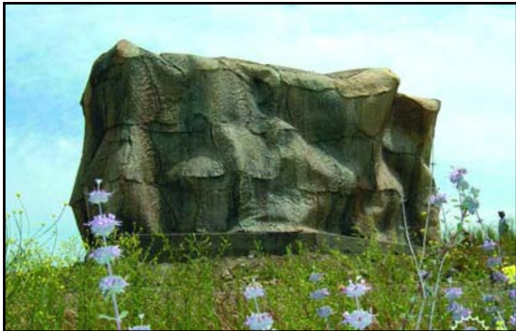
Figure-45. Baron Brothers' Nursery in Camarillo, CA. Antennas are located inside of the structure, which is made of a radio frequency transparent material. Dimensions of the structure are 25 feet wide by 12 feet high.
