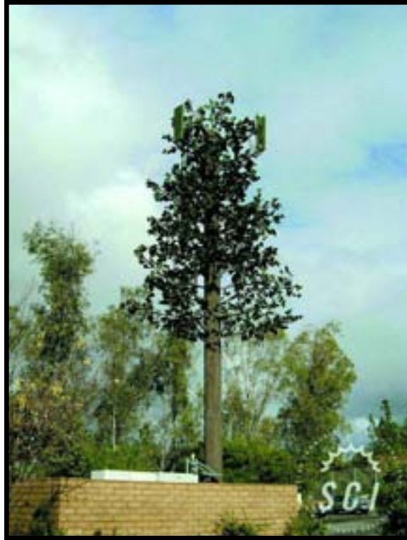
Figure-30. Pacifica Mormandie in Torrance, CA. The structure is 62 feet tall. Antennas are located at 55 feet agl.
