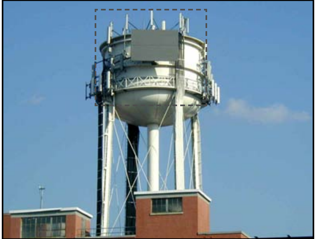
Figure-9. A passive microwave reflector is located at 652 Glenbrook Road in Stamford, CT. Photograph taken in December of 2006.
