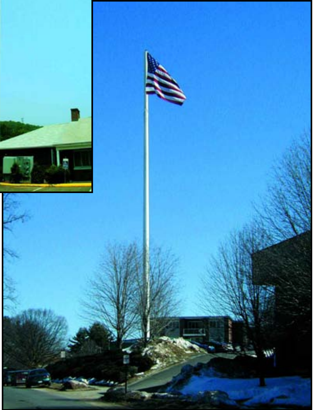
Figure-33. 985 Farmington Avenue in Bristol, CT. Antennas are located within the flagpole structure and equipment is at the base of the structure.
