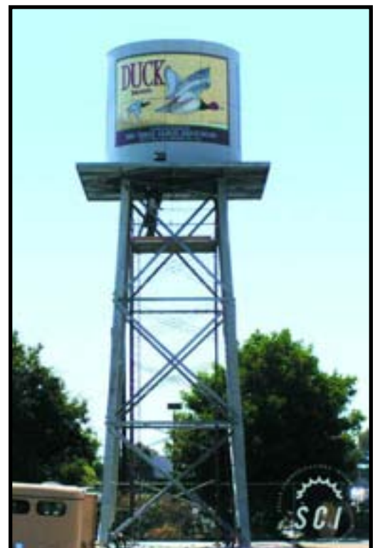
Figure-43. Via Verde in San Dimas, CA. The structure is 60 feet tall. Antennas are mounted within the water tank at 58 feet agl and 47 feet agl.
