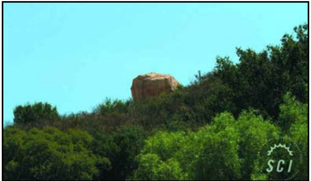
Figure-47. Rocky Peak Church in Chatsworth, CA. Antennas are located inside of the structure, which is made of a radio frequency transparent material. Dimensions of the structure are 11 feet 6 inches tall by 8 feet in diameter.
