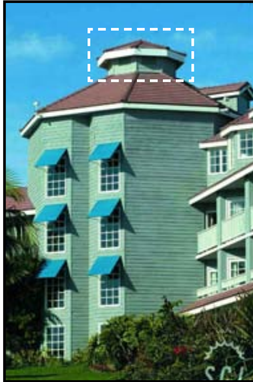
Figure-53. Lantern Bay in Dana Point, CA. The height of the structure is 54 feet 11 inches. The antennas are located at 50 feet 11 inches agl.
