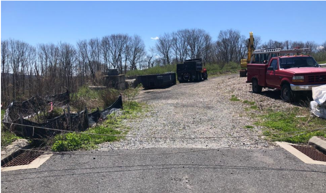
Before construction - Wetland 1 to left, surrounded by silt fencing
