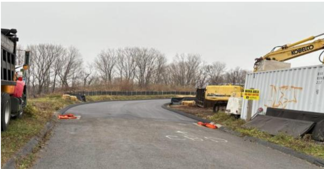
After construction - Wetland 1 location to left, beyond catch basin
