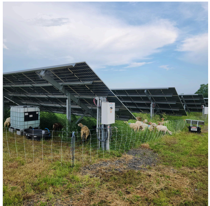
Right Above: Sheep grazing infrastructure - Water System, Electric fencing, Electric Fencing Charger
