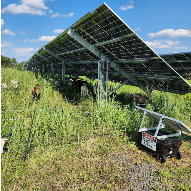
Left Above: Portable, Solar-Powered Electric Fence Charger
