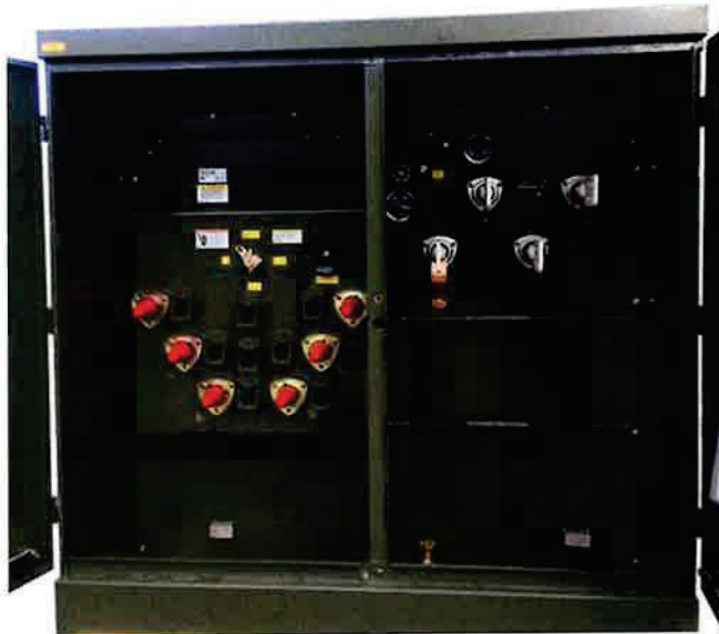
Fig 2. Three Phase Maddox Padmount Transformer
