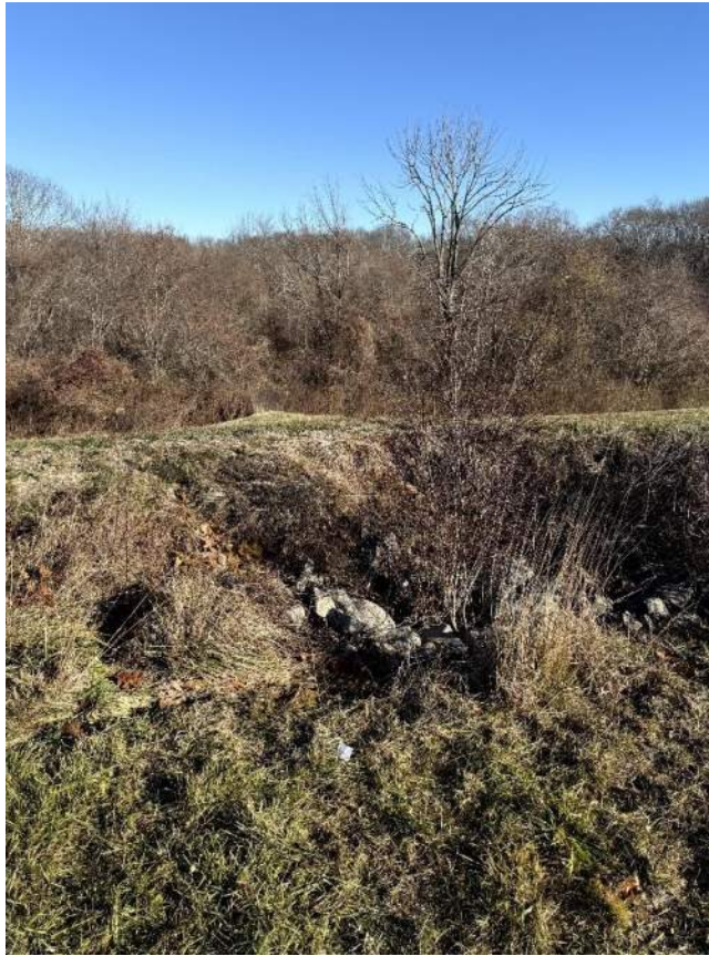
Photo 7: Existing stormwater control feature (18" CPP inlet) looking north. Forest edge in the background as well as the approximate location of agricultural soil areas.
