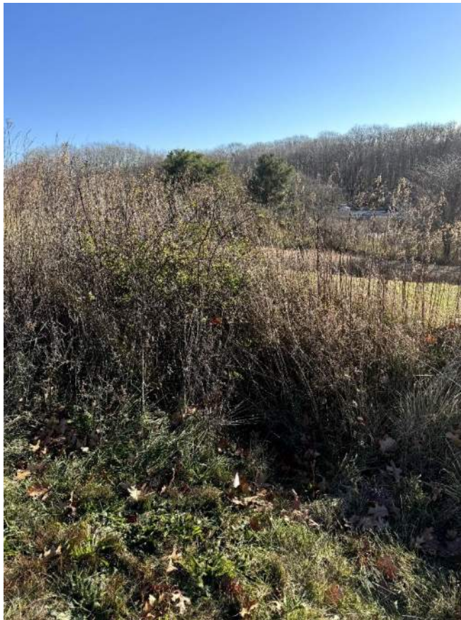
Photo 14: Existing stormwater control feature (15" CPP inlet) looking south towards I-95
