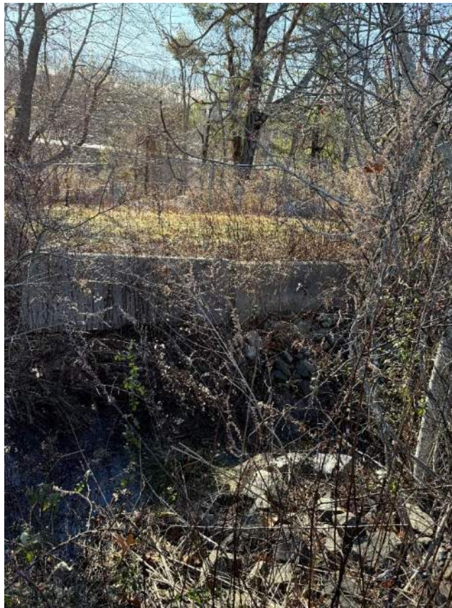
Photo 15: Existing stormwater control feature (15" CPP inlet) looking south towards I-95. This structure is located within the flagged wetlands adjacent to I-95.
