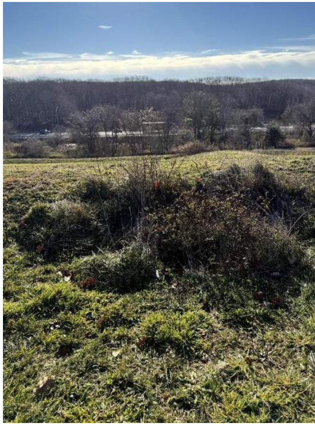
Photo 13: Existing stormwater control feature (15" CPP inlet) looking south towards I-95
