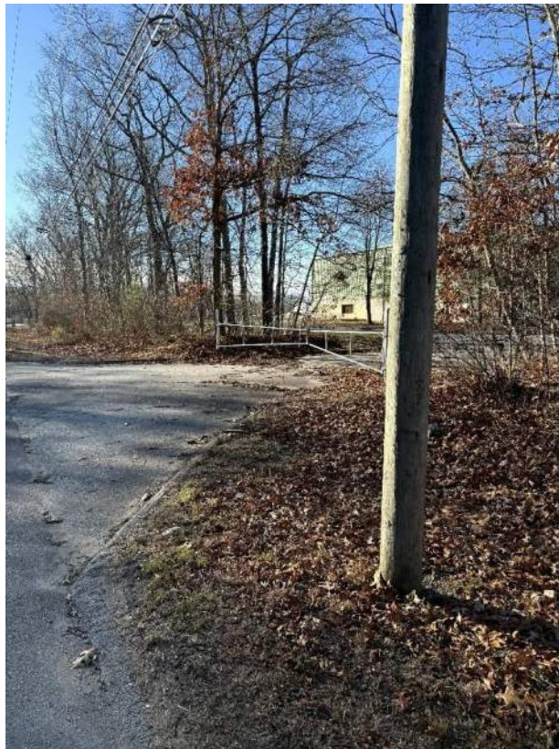
Photo 2: Point of interconnection. Existing Eversource Utility Pole #6249 adjacent to proposed site entrance along Flanders Road looking south.
