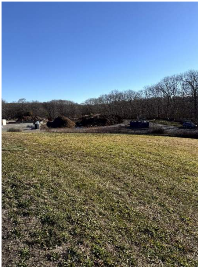
Photo 18: Sloping terrain of the landfill on the southeast side of the proposed solar array. Transfer station refuse in the background.
