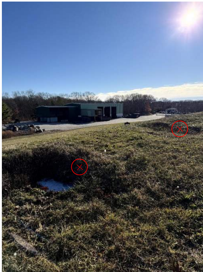
Photo 6: Existing stormwater control features (15" CPP) looking southeast.
