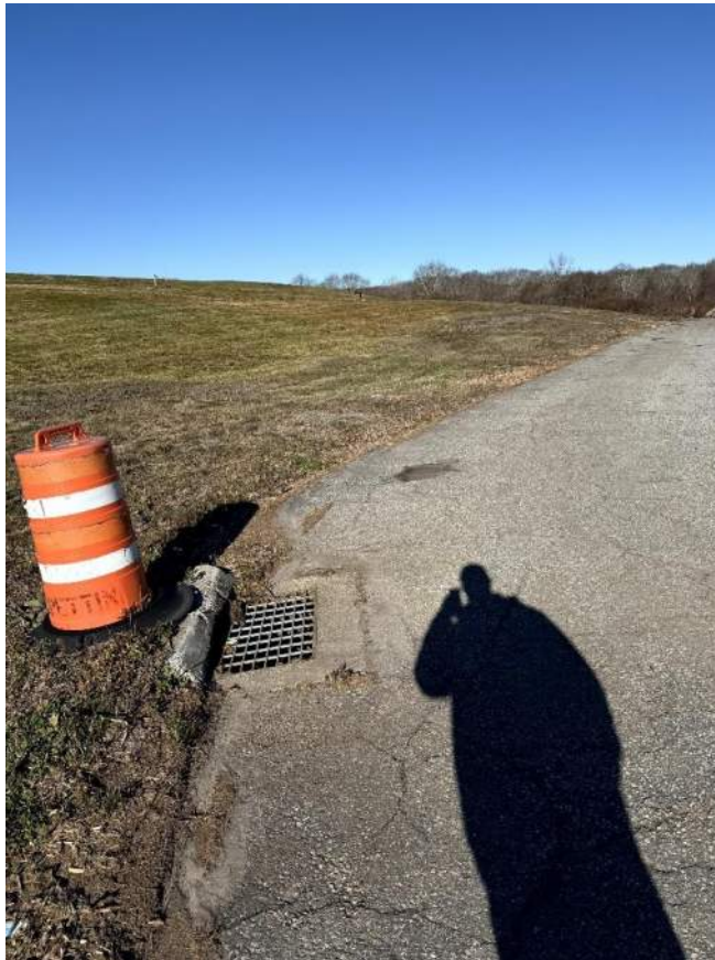
Photo 20: Existing stormwater catch basin located to the south of the proposed utility pad adjacent to the existing cell tower compound. Picture is looking north.
