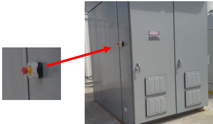
Tie Breaker Switchgear ( Site Electrical Disconnect )
