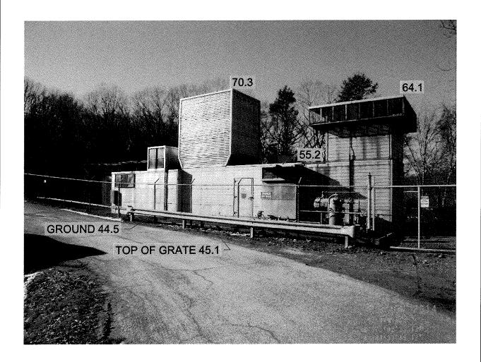
THE EXISTING VERTICAL PLANT DATUM IS NGVD1929. IT WAS CONFIRMED USING STATIC GPS OBSERVATIONS ON KNOWN SURVEY CONTROL, WHICH WERE POST PROCESSED USING OPUS AND CONVERTED FROM NAVD1988 USING U.S.G.S. CORPSCON SOFTWARE. THE OBSERVED ELEVATIONS AGREED WITHIN ~0.1 FEET.
