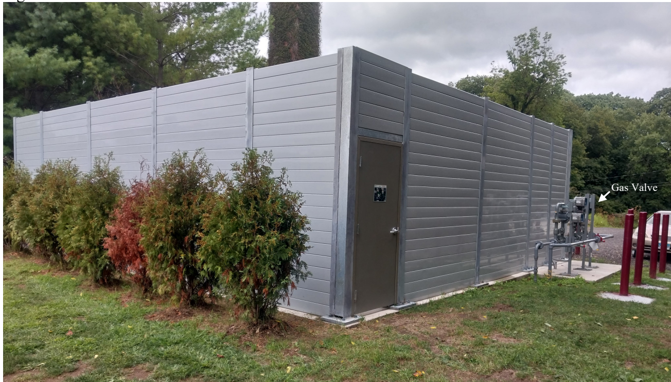
Figure 2. Photo of the Bloom Fuel Cell Noise Enclosure
