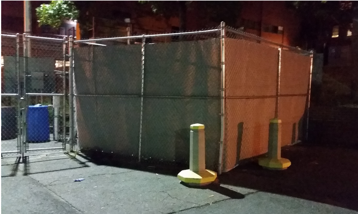
Figure 8. Eight Foot Fence Surrounding Doosan Cooling Module with Noise Treatment
