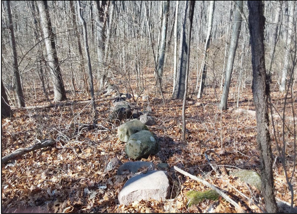
Photo 11. Overview photo of stone wall. Photo taken facing west.
