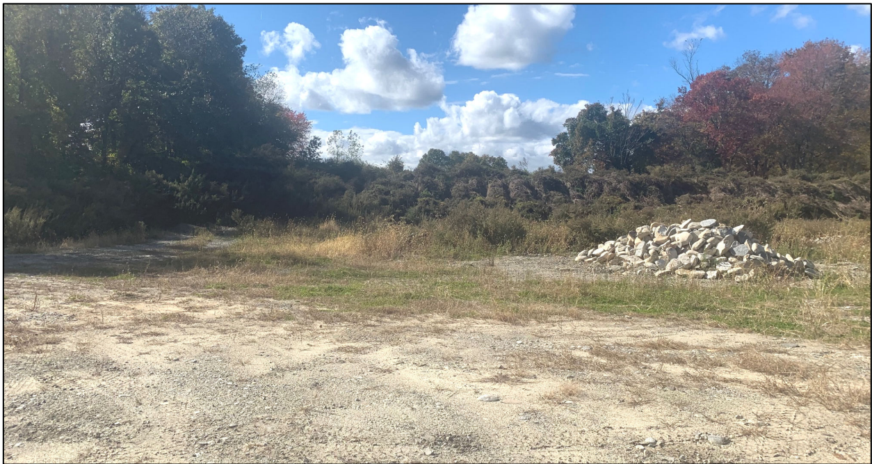
Figure 7: Southwest view of the staging area on the west side of the road, quarried out, leveled, and used for temporary storage of materials. Southwest of larger quarry area.
