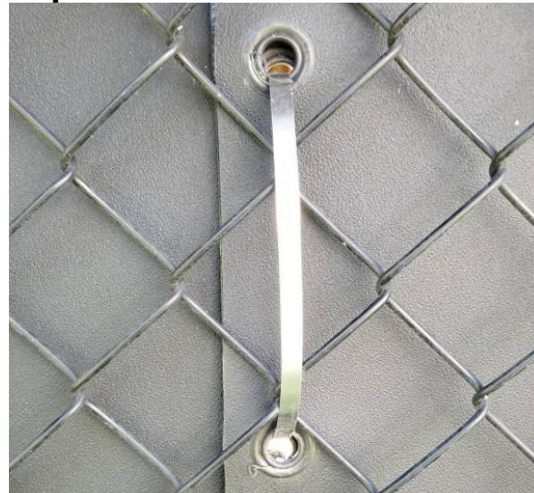
Overlap Seam – Chain Link Side Close Up
