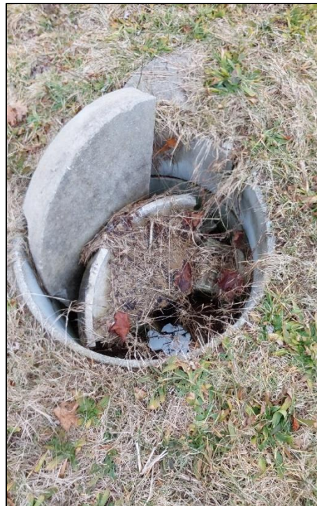
Photo 4. Close up of manhole in the facility area.
