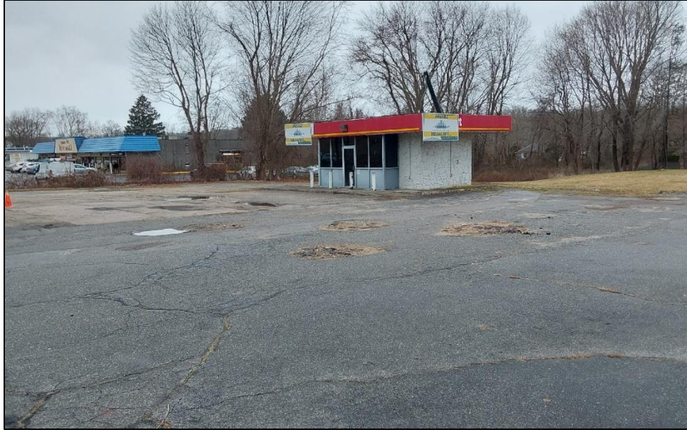
Photo 1. Overview photo from northeastern corner of the parking lot. Photo taken facing southwest.
