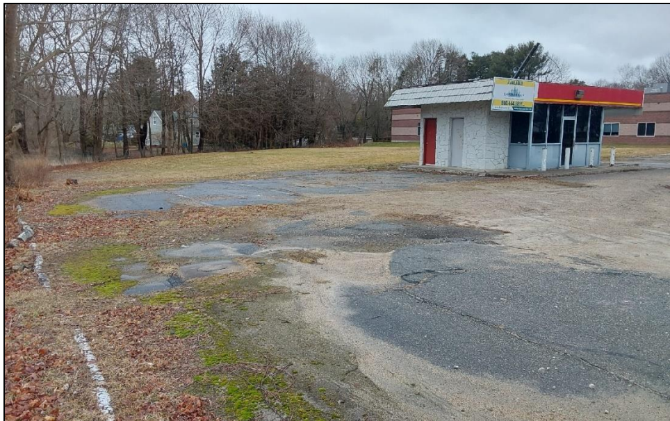
Photo 2. Overview photo from southeastern corner of the parking lot. Photo taken facing northwest.
