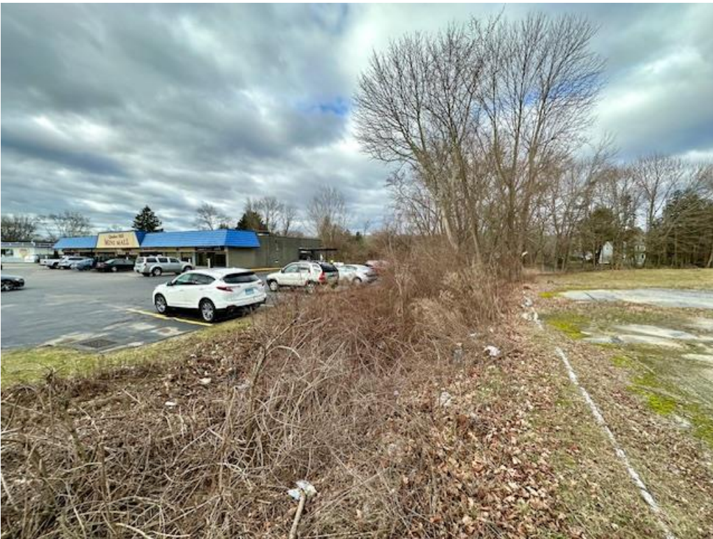
Photo 4: Existing Conditions of the Drainage Ditch Between 40 Norwich Road and 30 Norwich Road.
