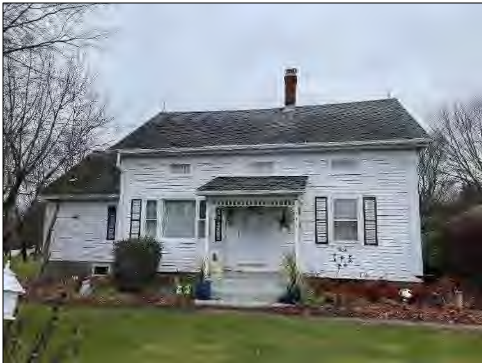
Photo 26. Overview of southeastern elevation of 341 Foster Street (Resource 50). Photo facing to the northwest.
