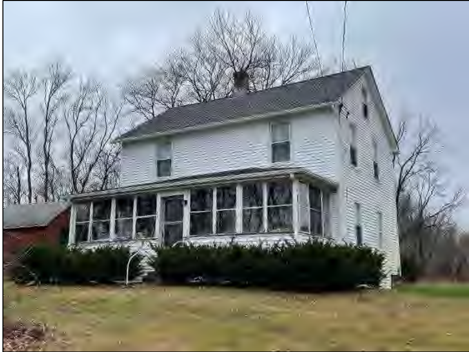
Photo 9. 3/4 of southeastern elevation of 255 Avery Street (Resource 7). Photo facing to the west.
