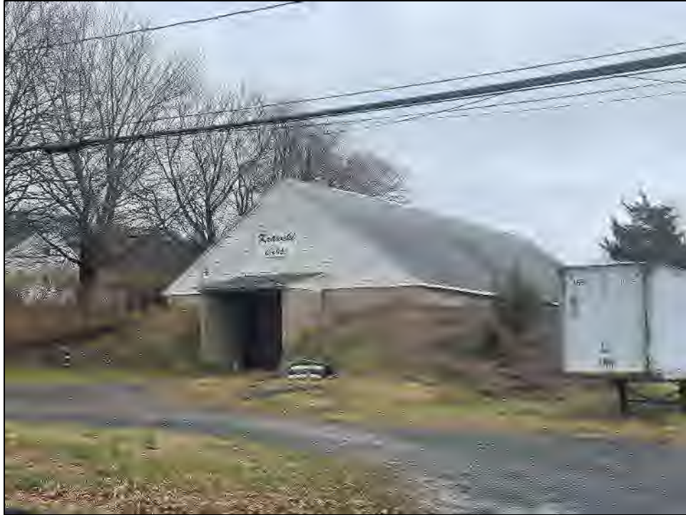
Photo 31. 3/4 view of northwestern elevation of R002 Foster Street (Resource 43). Photo facing to the northeast.
