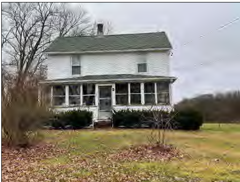
Photo 8. Overview of southeastern elevation of 255 Avery Street (Resource 7). Photo facing to the northwest.
