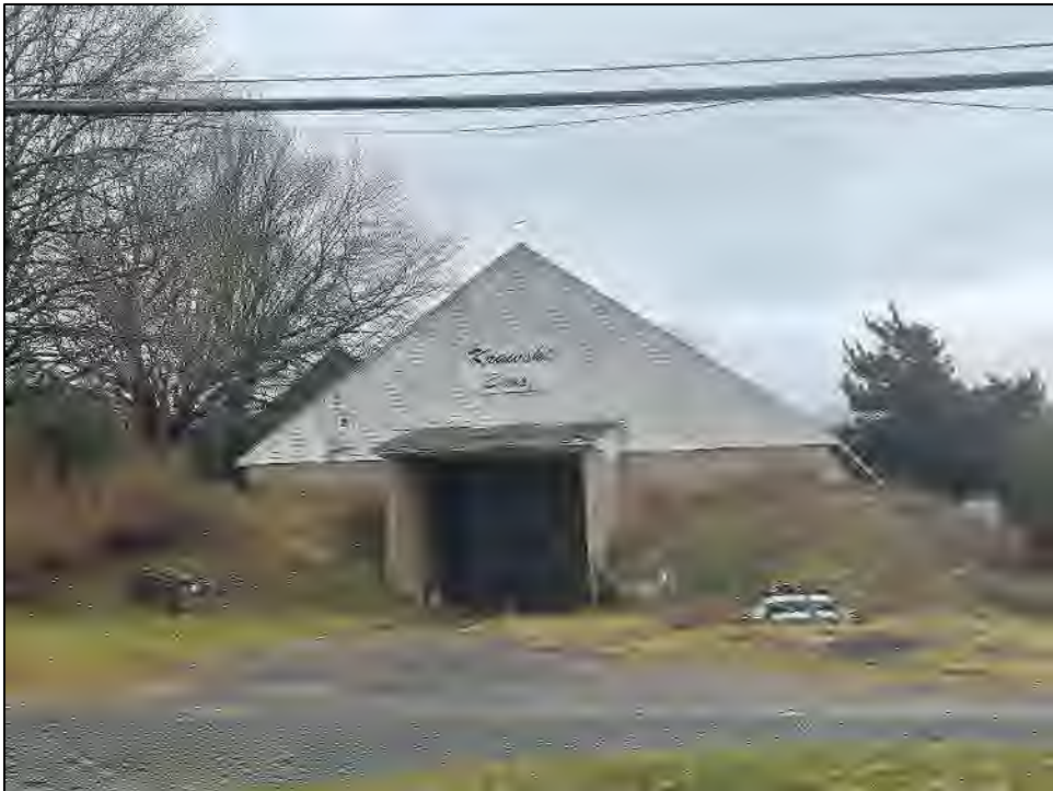
Photo 30. Overview of northwestern elevation of R002 Foster Street (Resource 43). Photo facing to the southeast.
