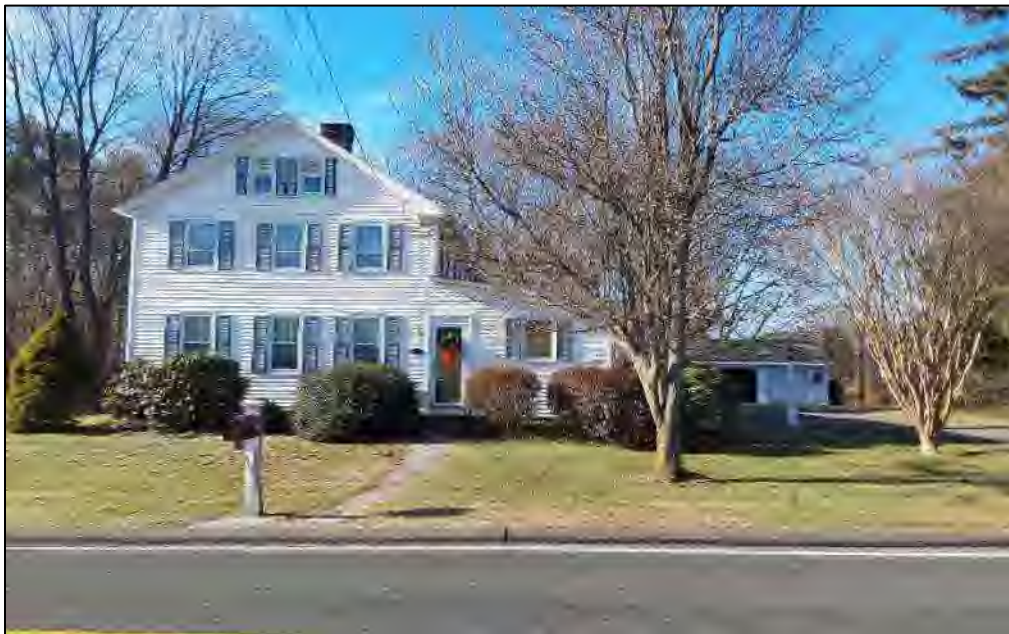
Photo 34. Overview of southeastern elevation of 179 Foster Street (Resource 48). Photo facing to the northwest.
