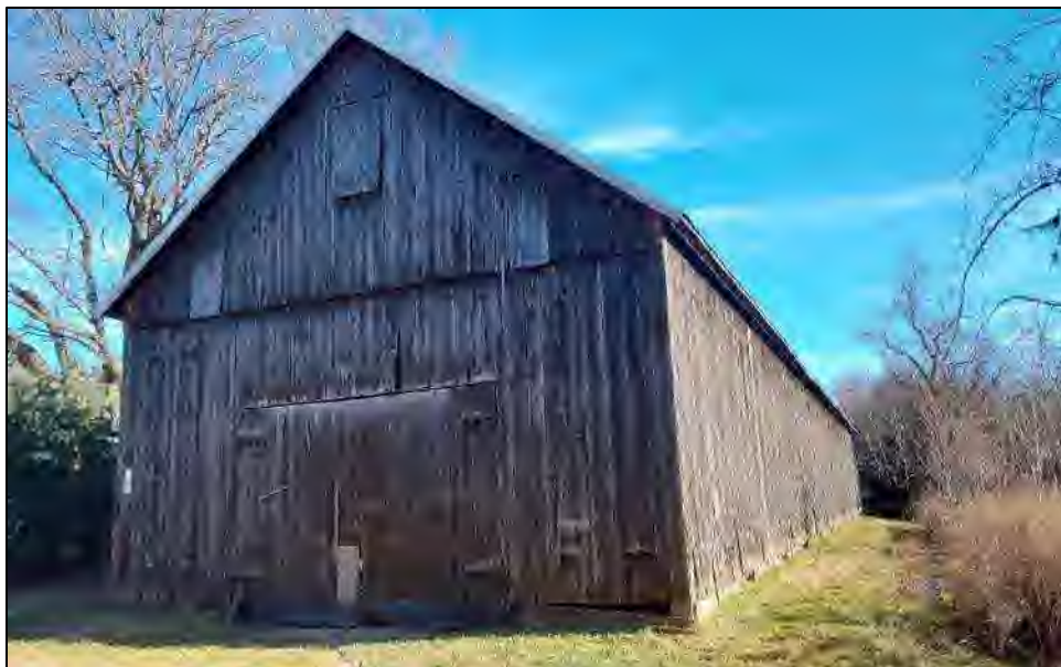
Photo 28. 3/4 view of northwestern elevation of 186 Foster Street (Resource 49). Photo facing to the southeast.
