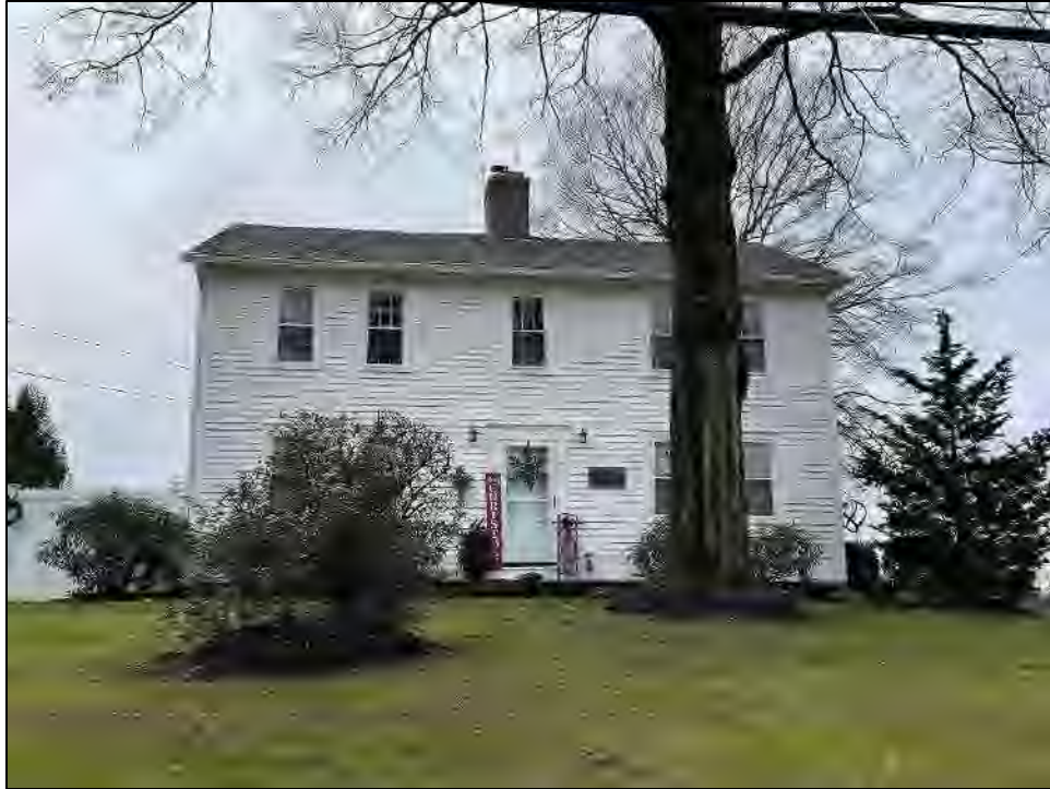
Photo 21. Overview of northwestern elevation of 90 Foster Street (Resource 45). Photo facing to the southeast.
