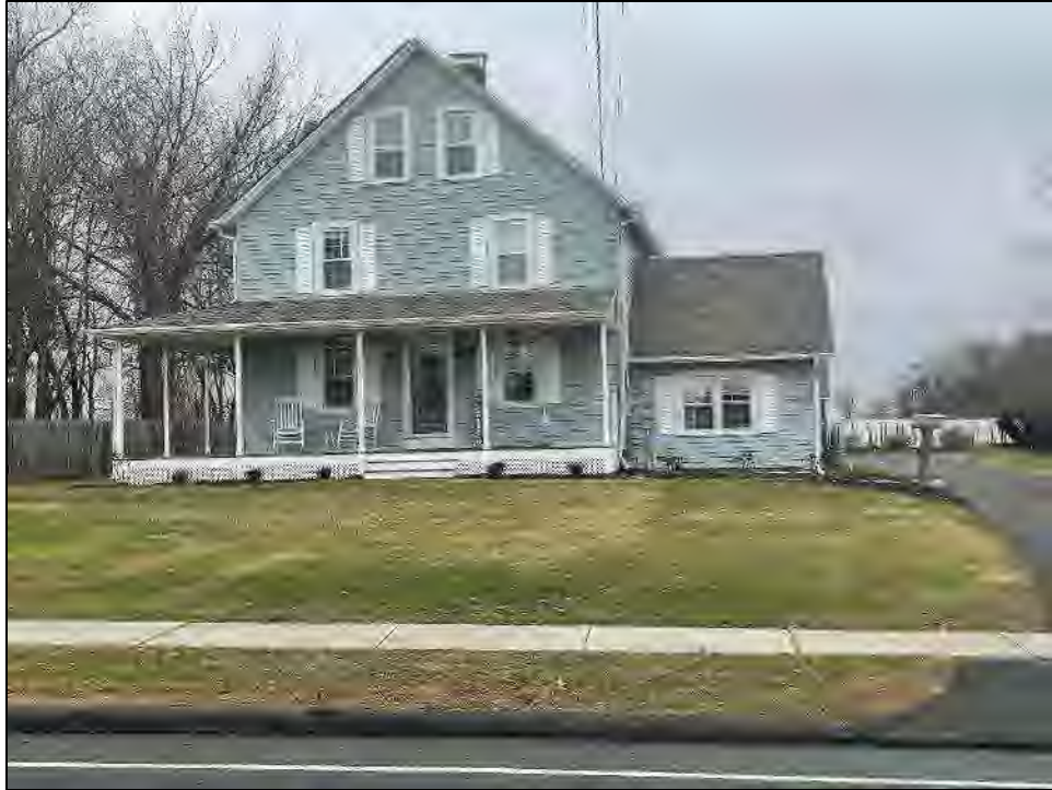
Photo 11. Overview of southeastern elevation of 229 Avery Street (Resource 6). Photo facing to the northwest.
