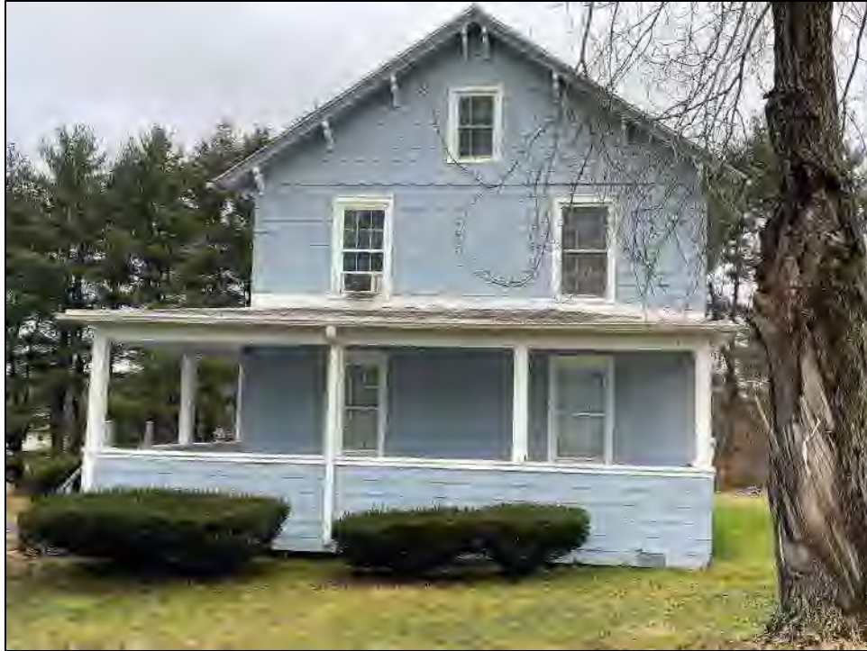
Photo 23. Overview of southeastern elevation of 117 Foster Street (Resource 46). Photo facing to the northwest.
