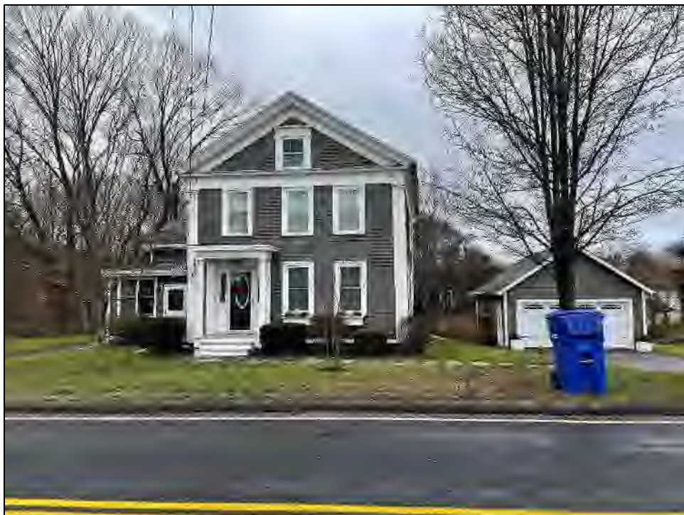
Photo 18. Overview of southeastern elevation of 63 Foster Street (Resource 44). Photo facing to the northwest.
