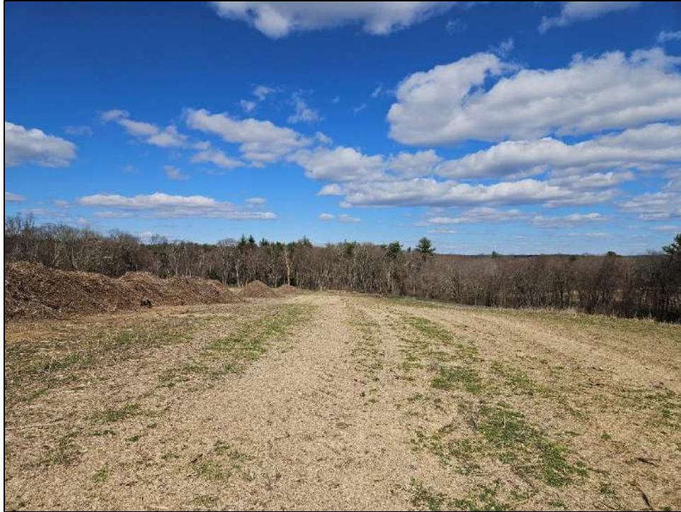
Photo 1. Overview of the western portion of the development area. Photo taken facing to north.
