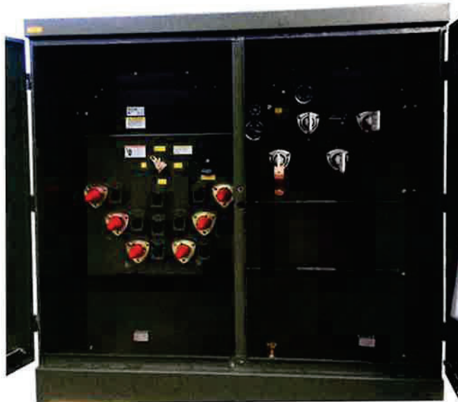
Fig 2. Three Phase Maddox Padmount Transformer
