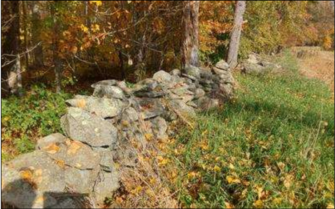
Photo 13. Overview of dry laid stone wall along western boundary of project parcel. Photo facing northeast. Note stone wall runs northeast to southwest.
