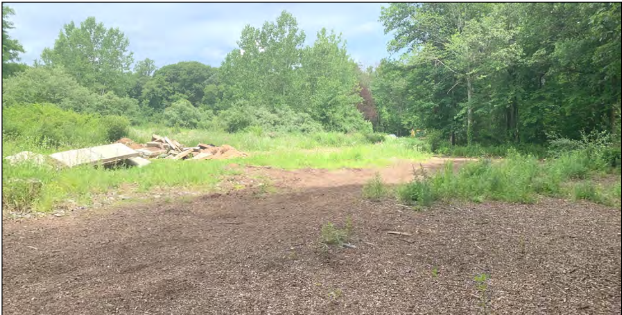
Figure 7: North view of the project area, demolished remains of the former industrial building at left, narrow wooded strip of land at right.
