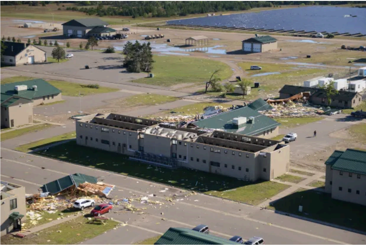
Multiple buildings on Camp Ripley, including those used for housing, training and maintenance, received damage during a late-night storm and small tornado that moved through Morrison County on Sept. 7, 2016. (Photo courtesy of Minnesota National Guard: SSG Anthony Housey)
