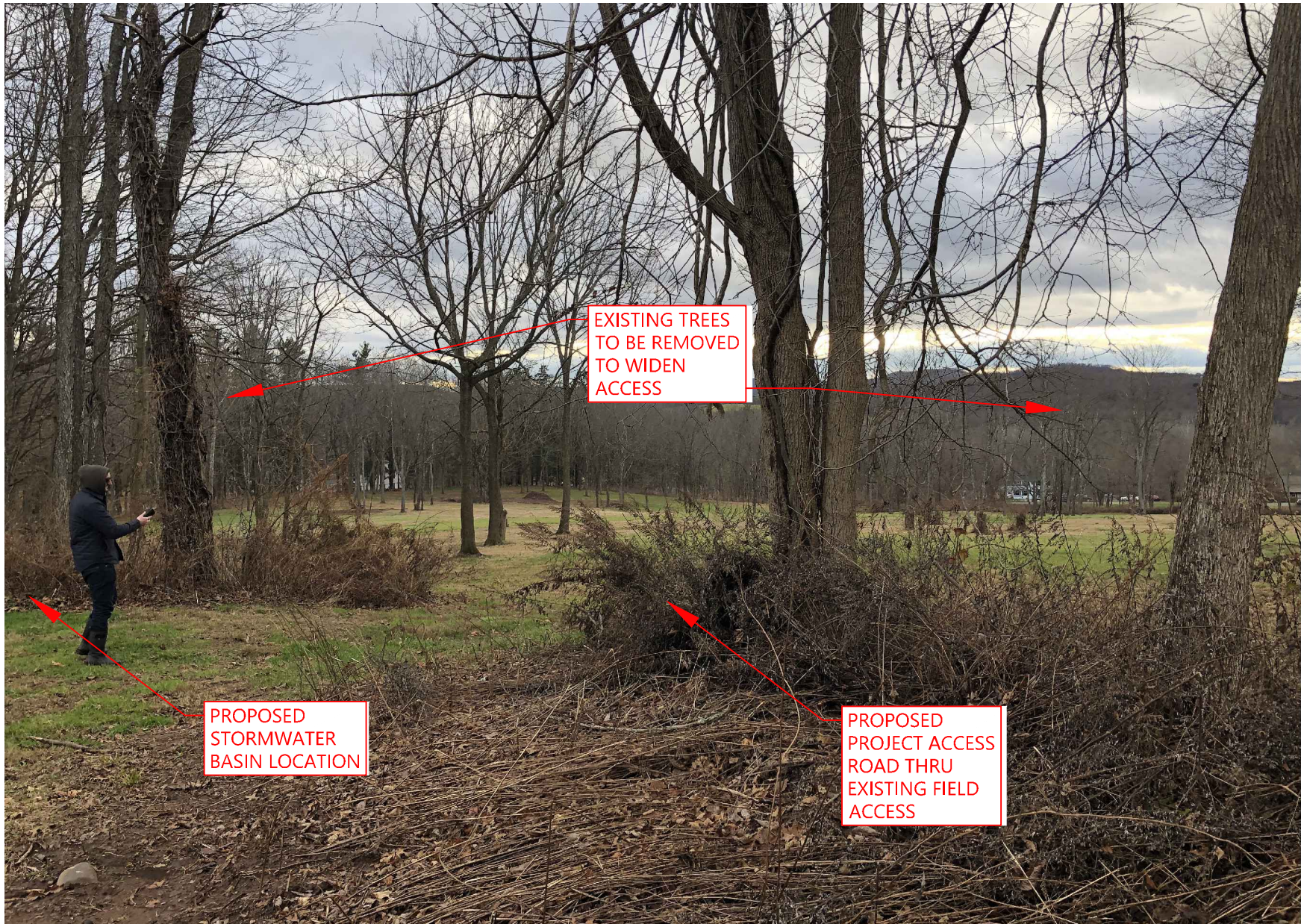
Photo 4 Existing Access; Stormwater Basin 2B Location
