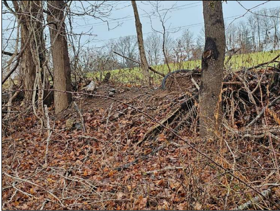
Photo 25. Overview of push pile against Stonewall 2, Segment 3. Photo taken facing to north.
