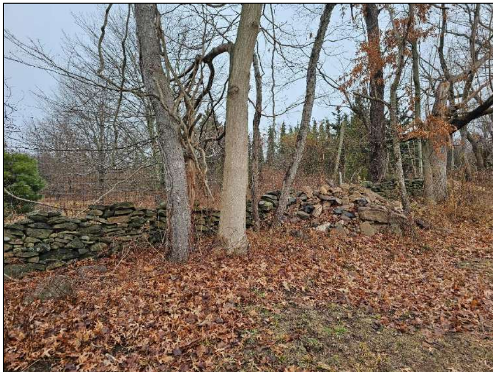
Photo 20. Overview of Stonewall 2, Segment 1 with evidence of pushpiles. Photo taken facing to east.
