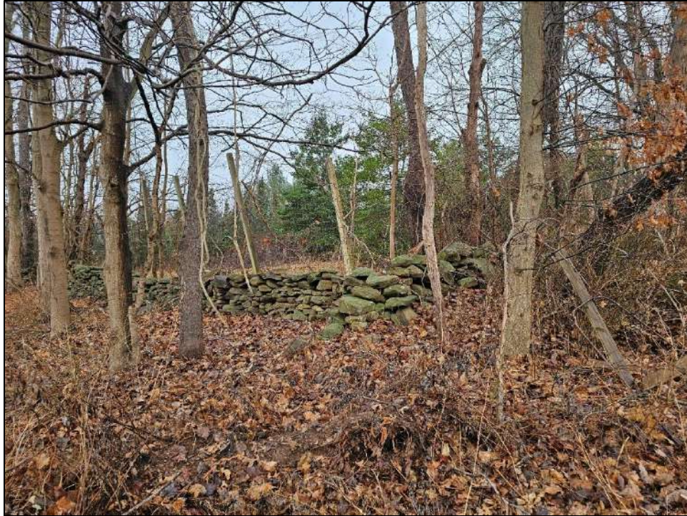
Photo 21. Overview of the intersection of Stonewall 2, Segments 1 and 2. Photo taken facing to northwest.
