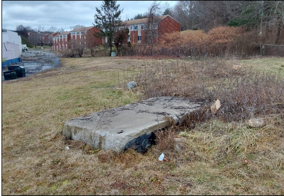
Photo 3. Overview photo of a concrete pad within the project parcel. Photo taken facing northwest.
