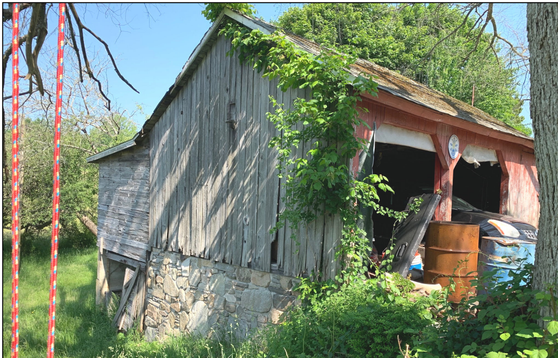
Figure 7: Northwest view of south end of garage, showing stone foundation.
