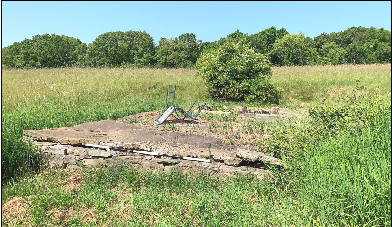
Figure 8: Southwest view of late historic foundation and concrete slab of former structure located just east of project area, which occupies farm field in background.
