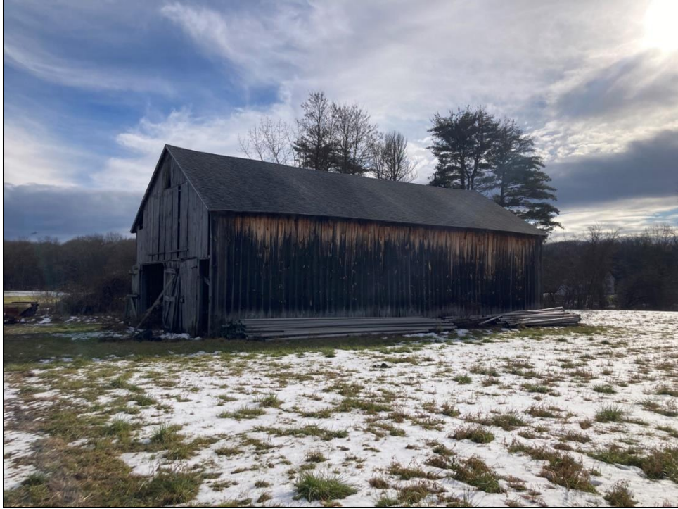
Photo 13. 3/4 view of north elevation of Structure 1. Photo facing to the southeast.
