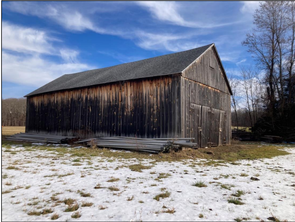
Photo 14. 3/4 view of south elevation of Structure 1. Photo facing to the northeast.
