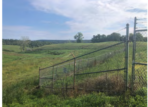
Photo 16: Looking northeast between metal hydroxide sludge and municipal waste fill areas.
