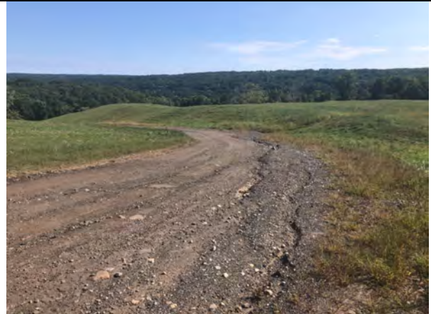
Photo 4: Looking northeast from top of landfill along main access road.
