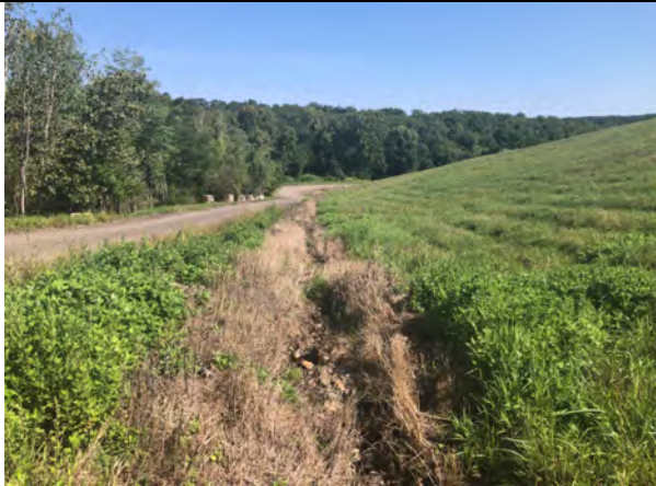
Photo 3: Looking north down drainage swale along main access road.
