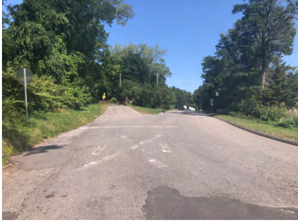
Photo 1: Access to former landfill from Vista Drive.
