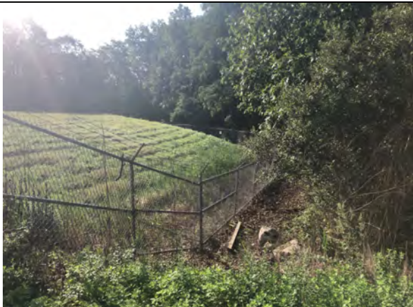
Photo 17: Looking southeast along control fence of metal hydroxide sludge area.
