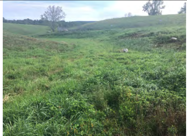
Photo 10: Looking northeast between metal hydroxide sludge and municipal waste fill areas.
