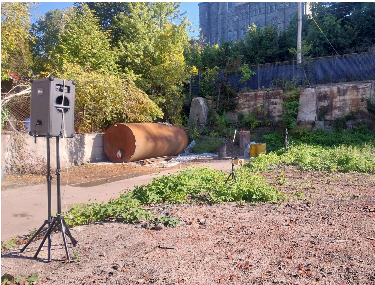
Figure 3. HiAxiom North Cooling Module Location Looking East at North Main Street
