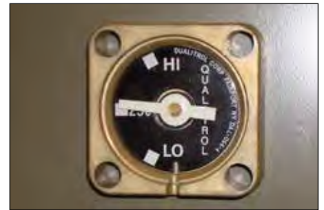
Figure 5. Liquid level gauge.
