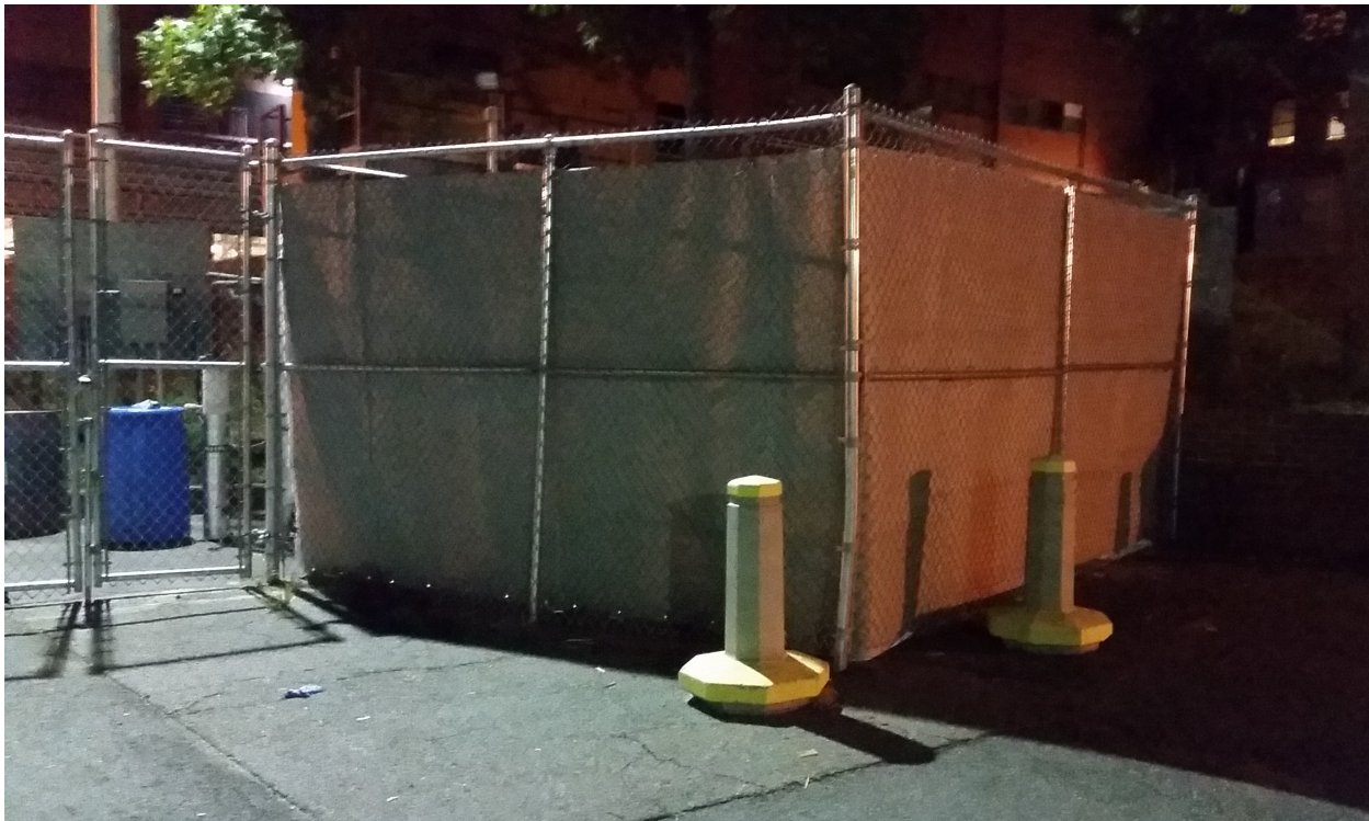
Figure 7. Eight Foot Fence Surrounding a Cooling Module with Noise Treatment
