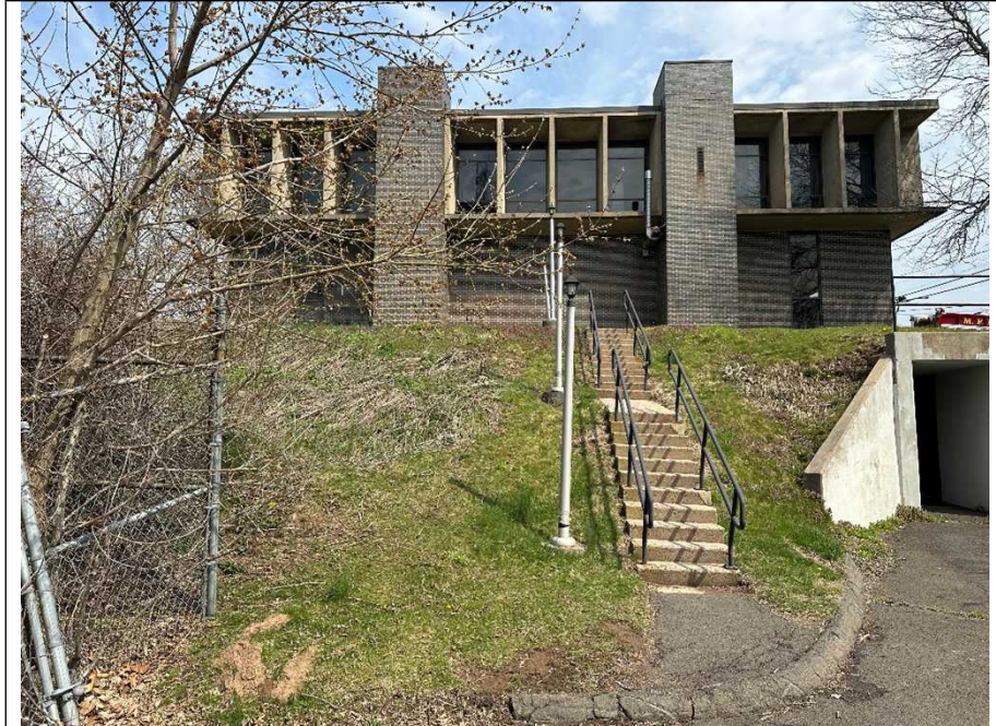
5. View from the proposed pole, facing north.
