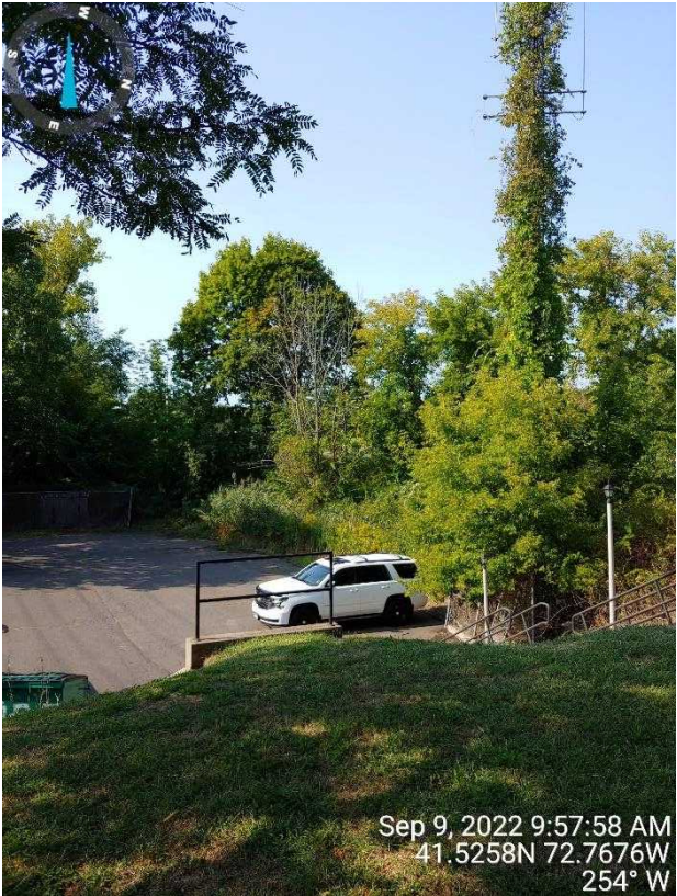
1. Fire Station Parking Lot and wetland (facing away from station building) with vine-covered communications tower
