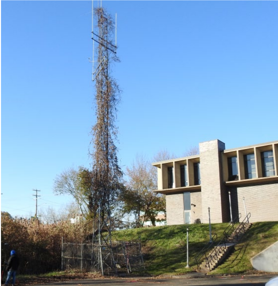
Figure 1 – Existing Municipal Self-Supporting Lattice Tower.
