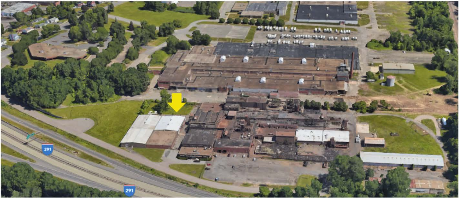
Aerial View - Battery system location indicated by yellow arrow
