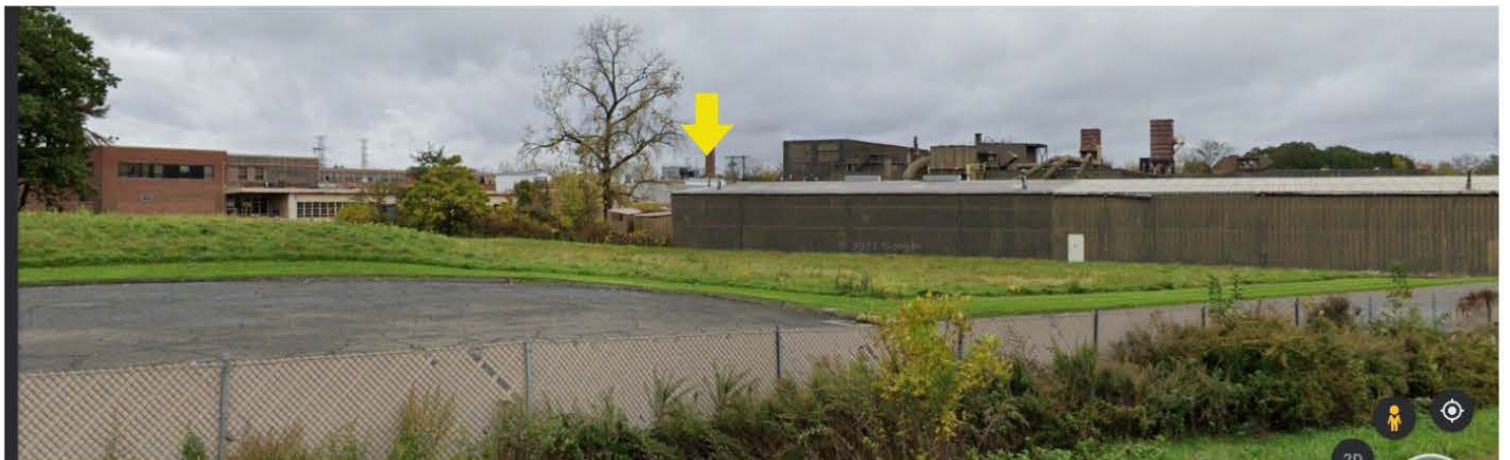
Ground View from I-291 Off-Ramp - Battery system location behind building.
