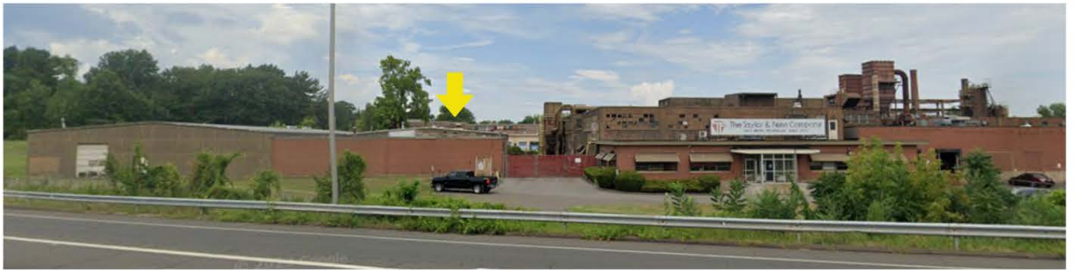
Ground View from I-291 - Battery system location behind building
