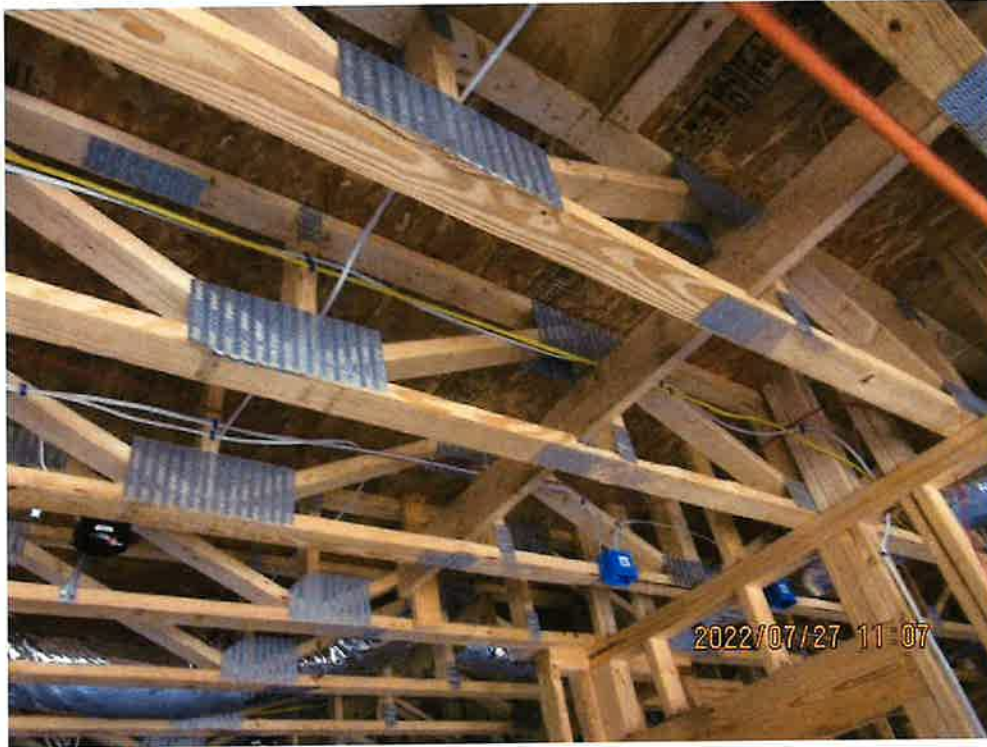
Photo 3: Sample photo illustrating the existing roof construction.
