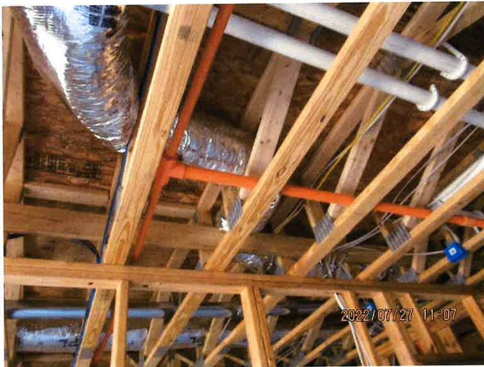
Photo 4: Sample photo illustrating the existing roof construction.
