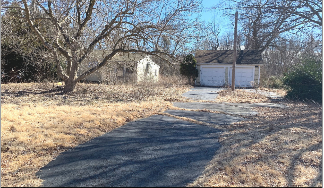
Figure 6: East view of the house and garage at 428 Bethmour Road.
