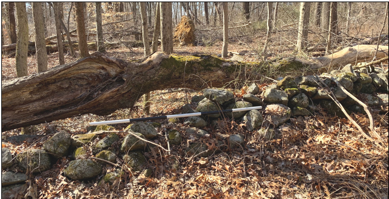
Figure 9: Southwest view of stone wall alignment in the wooded section of the project area.
