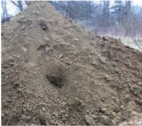
Bottom of test pit at 4.5 feet. Pictures showing soil strata at Test Pit 1
