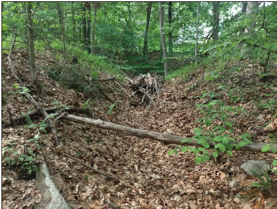
Photo 4. Drainage ditch located in the western portion of the sensitivity area in the Project area. Photo facing south.
