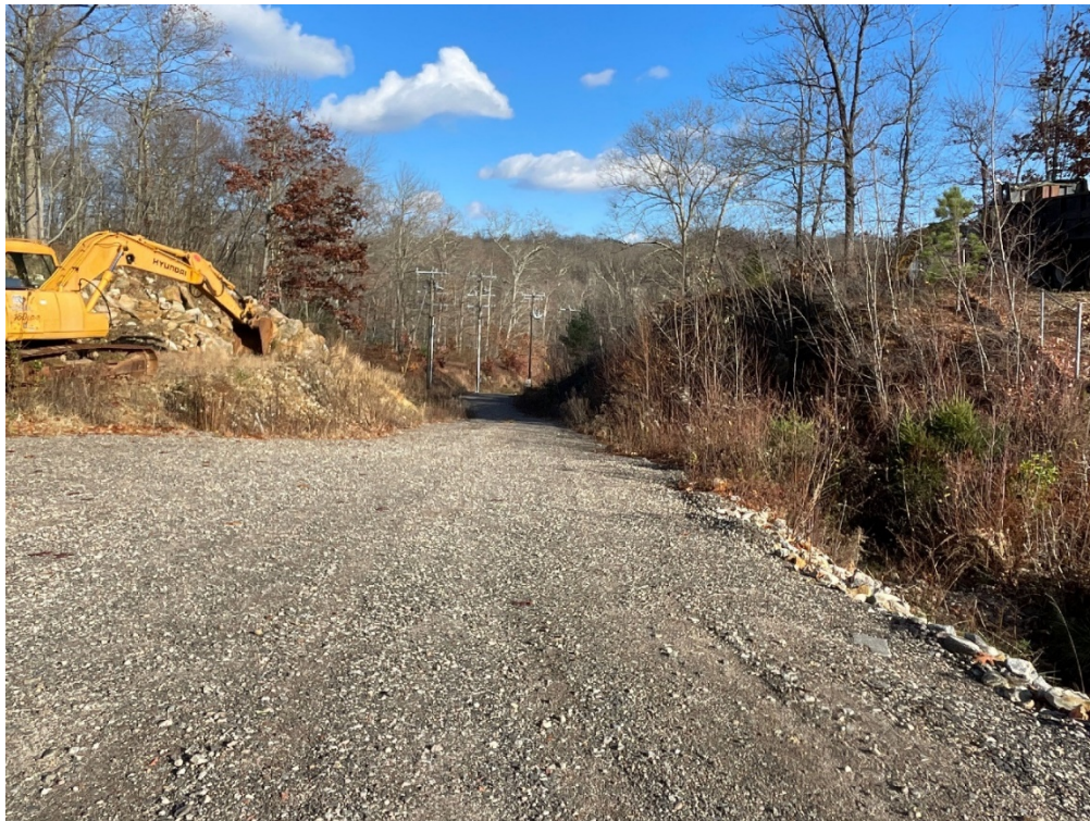
Access drive, November 17, 2022.
